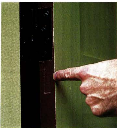
Full mortises are characteristic of pre-1860s frame-and-panel doors. In this construction method, the tenon extends all the way through the stile for maximum support. Note the scalloped surface of the door, the result of surface planing.
