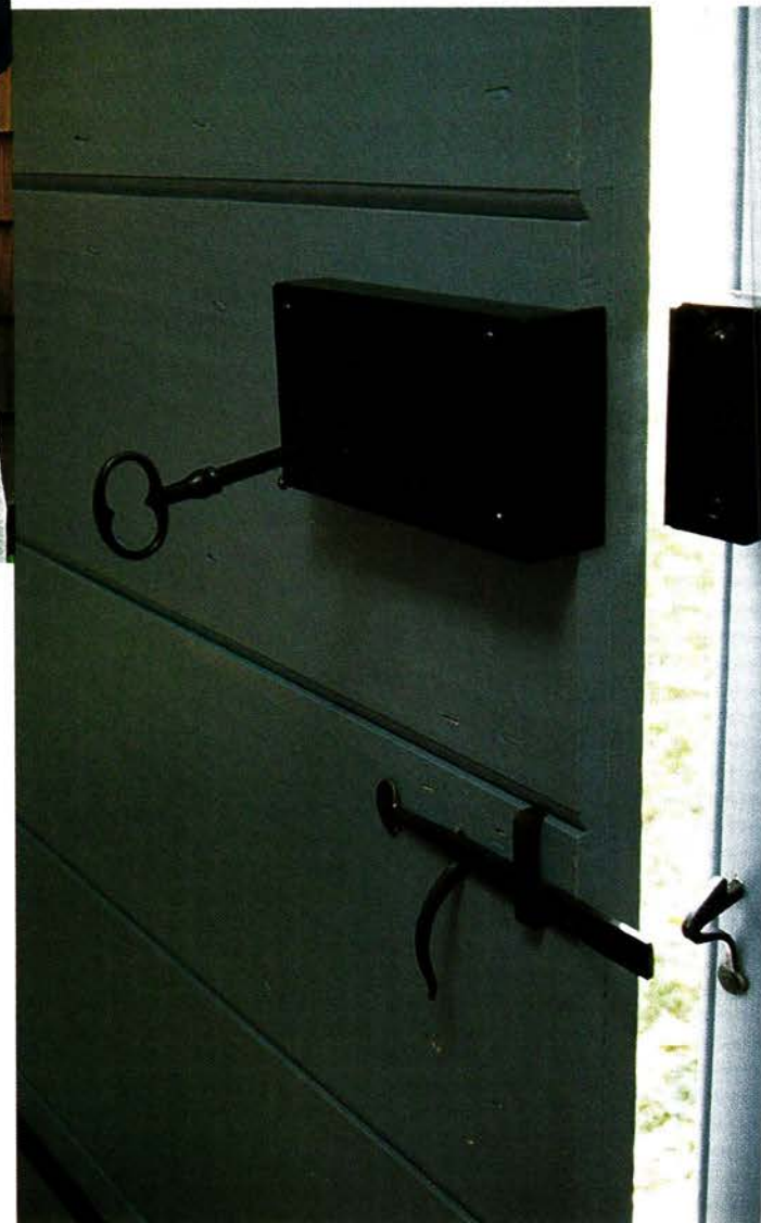
Above: Beyond scraps of 19th century newspaper still pasted to the surface, the batten door face shows the telltale metal loops of the clinched nails that hold it together. Below: Inside, each batten of the reproduction door half-laps the next in a shiplap joint. The thumbnail moulding copies the original, as do the thumbblatch and iron box lock.
