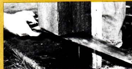
10" rotted bottoms of these load-bearing columns...
