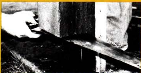
10" rotted bottoms of these load-bearing columns...
