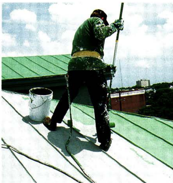
Water-based technology streamlined liquid membrane application to little more than product and roller. Basically sound roofs may require only primer and wearing coat.
