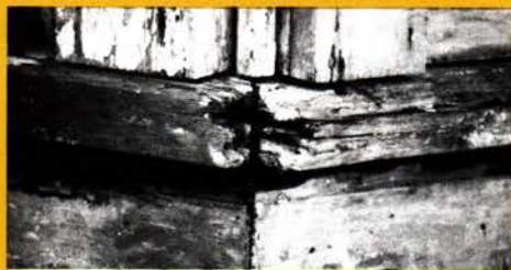
This rotted – and irreplaceable – woodwork...
