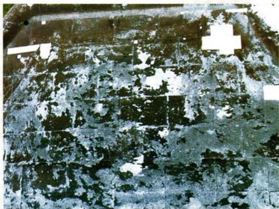
Left: Preparing the neglected terne metal roof meant wire-brushing off all loose paint and rust, and patching with new sheet metal (white areas in photo). Bottom left: Unrolling the fabric into the wet primer is one way to saturate the weave quickly. Below: The top layer holds the color and should be recoated every few years.
