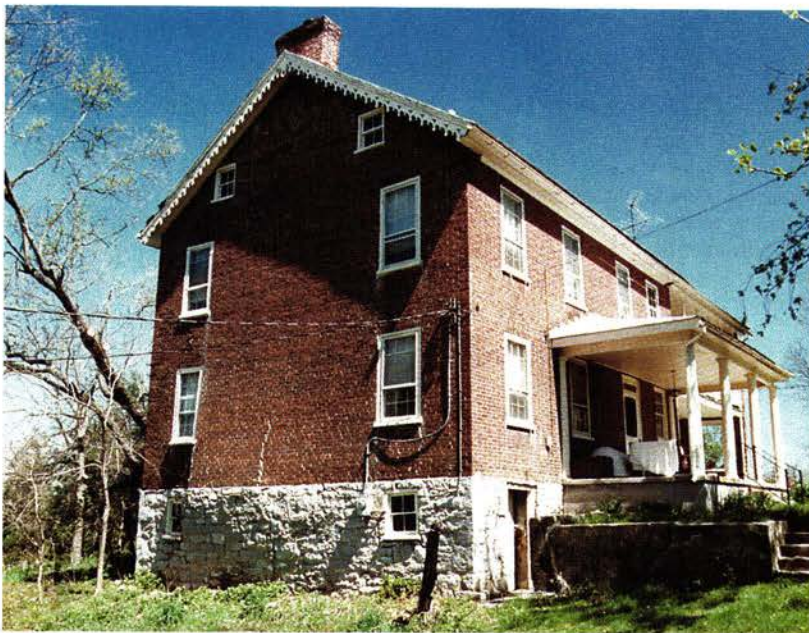
Deep shadows on the stone foundation show how far the wall had bellied by April of 1999—fractions of an inch away from total collapse.
