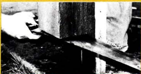
10" rotted bottoms of these load-bearing columns...
