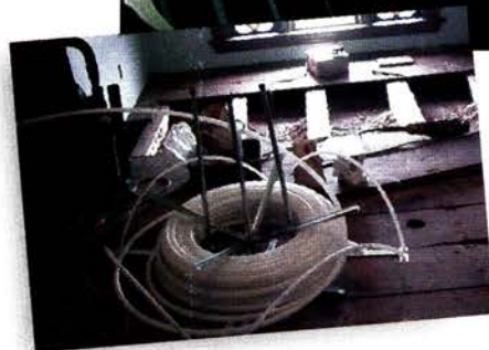
Top, left to right: Polyethylene tubing ready to go under the floorboards. A workman slides a radiator through the upper hall, while a crane delivers another to the second storey. Bottom: Glenn and Gail found time to do up a period bathroom.
