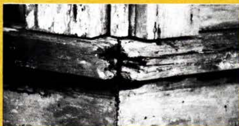
This rotted – and irreplaceable – woodwork...
