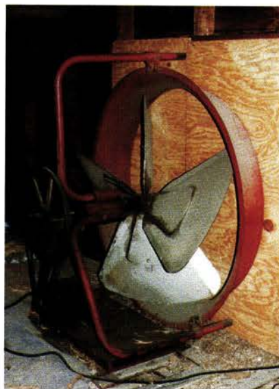
Top: Look for oil caps near the motor bearings (center in photo) and on the blade shaft. Above: Plywood or insulation blocks heat loss through the vent in winter.
