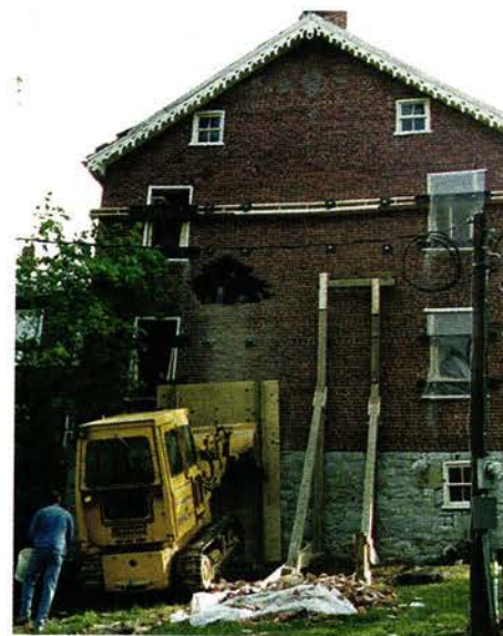
Above: Outside, timber shores and an earthmover stabilize the bulge while dismantling begins. Below: Inside, stud-walls and rods carry the floor and roof loads.
