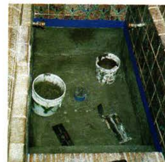
Clockwise from left: Two score marks on the tile wall separate what's to be sacrificed from what's to be saved. The new shower pan, an impervious membrane, gets the water test. Diamond lath sets the stage for the scratch coat and dry-pack mud bed.
