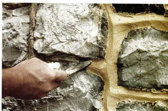
Top: Using a mason's "pastry bag" Paul Wade fills joints in the dressed-limestone foundation with finish mortar. Above: To match the inverted-V pointing, he sculpts the mortar with a small trowel. The new mortar will weather to historic colors. Left: A stock item, the bag is faster for filling irregular joints than pushing mortar off a trowel.
