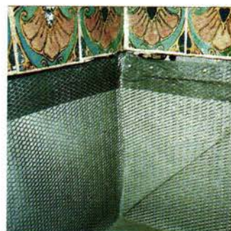
Clockwise from left: Two score marks on the tile wall separate what's to be sacrificed from what's to be saved. The new shower pan, an impervious membrane, gets the water test. Diamond lath sets the stage for the scratch coat and dry-pack mud bed.
