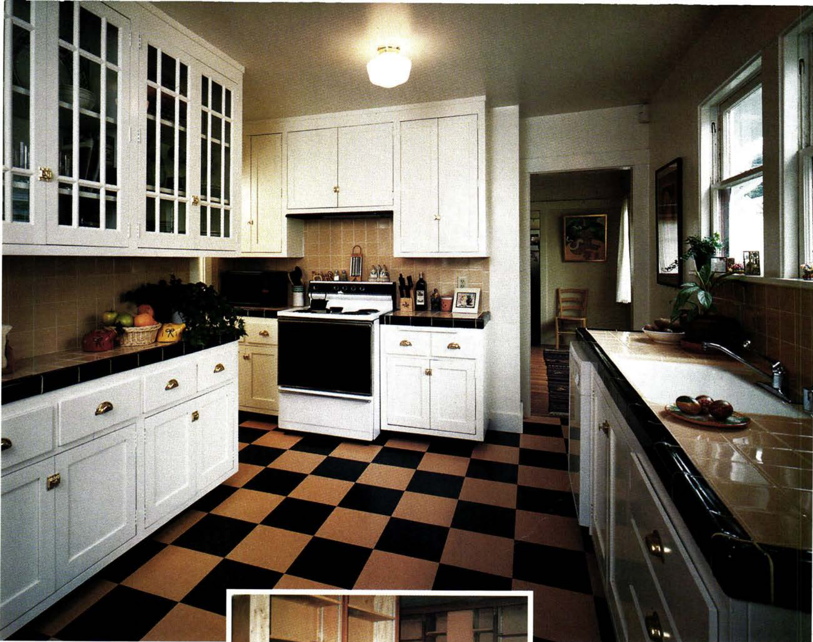
Keeping old kitchen casework (inset), but adding newly milled flat-panel doors, tile countertops, and fresh paint enhances value at low cost. Moulding patterns for the glazed upper cabinets come from originals in the dining room (previous page).
