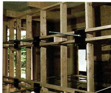
Above: Outside, timber shores and an earthmover stabilize the bulge while dismantling begins. Below: Inside, stud-walls and rods carry the floor and roof loads.
