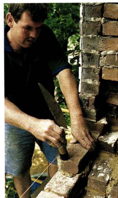
Above: Paul Wade prepares to set a brick with one hand as he "butters-up" the course with mortar using his other. Left: He taps each brick flush with a string line that marks correct wall position. Far left: Steve Fox adjusts each mortar joint so new brickwork will meet the old without resorting to partial bricks. In the background, note the massive gap between the plaster lath and bulging masonry—nearly equal to the thickness of the three-brick wall.
