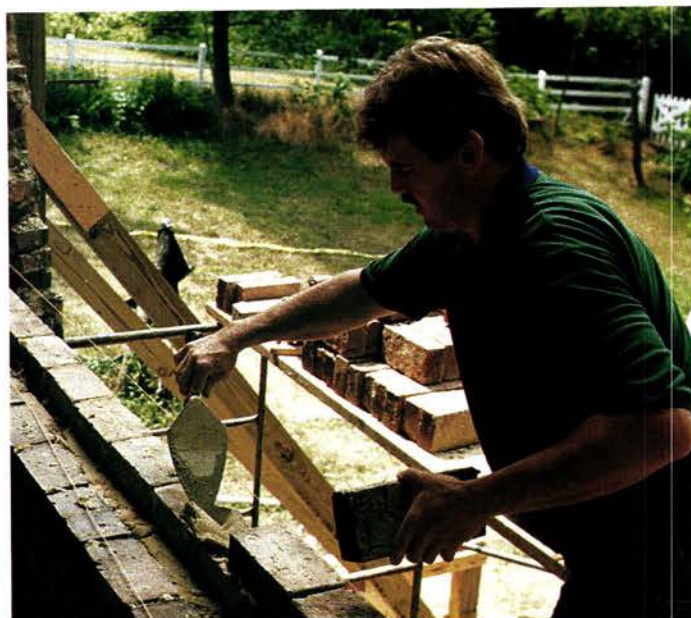
Above: Paul Wade prepares to set a brick with one hand as he "butters-up" the course with mortar using his other. Left: He taps each brick flush with a string line that marks correct wall position. Far left: Steve Fox adjusts each mortar joint so new brickwork will meet the old without resorting to partial bricks. In the background, note the massive gap between the plaster lath and bulging masonry—nearly equal to the thickness of the three-brick wall.
