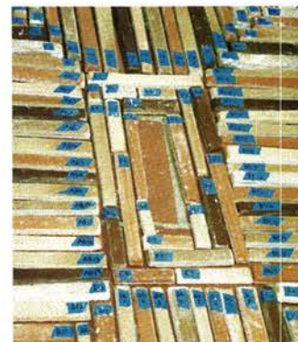
Top: Although the glazed floral tiles on the shower risers had to be replaced with plain, bisque-colored tile, the more visible tile on the treads mimics the original look. Above: Doty lays out the pattern and numbers each tile. Left: The new shower floor is a dead ringer for the old one (opposite, far left).
