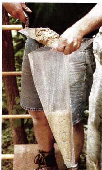
Top: Using a mason's "pastry bag" Paul Wade fills joints in the dressed-limestone foundation with finish mortar. Above: To match the inverted-V pointing, he sculpts the mortar with a small trowel. The new mortar will weather to historic colors. Left: A stock item, the bag is faster for filling irregular joints than pushing mortar off a trowel.
