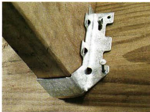
Top: Stainless steel siding nails. Above: Hot-dip galvanizing (left) and electrocoating. Left: Galvanized hanger nail.
