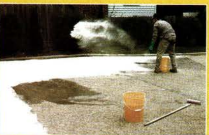
Grit being applied to restored driveway
