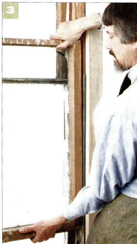
With one stop off, there's enough clearance to lift and angle the sash out of the window (3). Before removing the sash, secure the weight with a knot or clamp (4); the cord end can easily pop out of the sash stile (see arrow, above).
