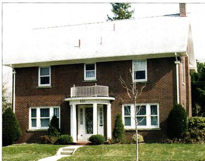
Replacing the iron railing atop this semicircular entry porch would restore the featured part of the Colonial Revival house. Inset: typical balustrade details from 1930.
