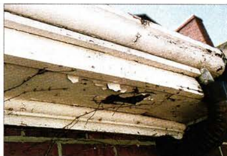
Clogged gutters also retain moisture that destroys troughs, such as in the wood gutter, causing paint failure and wood rot at eaves and walls.
