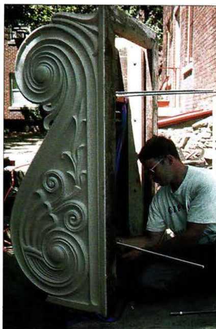
Before rehanging the console with threaded rods, Ted Robinson reinforced the heavy plank frame.
