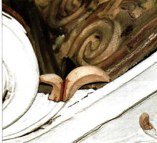
I attached the new elements with epoxy and nails, then bridged voids with epoxy filler.
