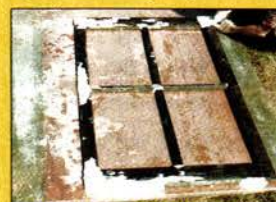
Antique window sash is salvaged, consolidated with LiquidWood and rebuilt with WoodEpox .
