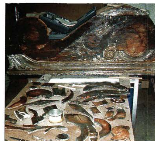
Saturating the console surface and relief elements with epoxy consolidant added integrity to the wood.
