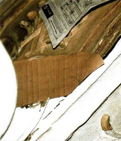
To carve missing elements I transferred the designs from historic drawings to cardboard.
