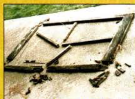
Antique window sash is salvaged, consolidated with LiquidWood and rebuilt with WoodEpox .
