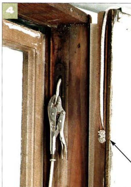
With one stop off, there's enough clearance to lift and angle the sash out of the window (3). Before removing the sash, secure the weight with a knot or clamp (4); the cord end can easily pop out of the sash stile (see arrow, above).
