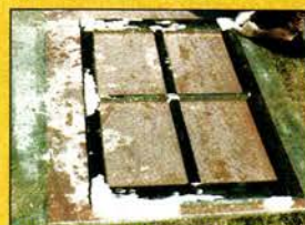
Antique window sash is salvaged, consolidated with LiquidWood and rebuilt with WoodEpoxy .
