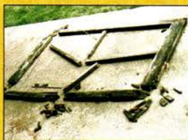
Antique window sash is salvaged, consolidated with LiquidWood and rebuilt with WoodEpoxy .
