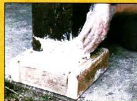
Rotted & infested base of a loadbearing column is completely sawed off and replaced with WoodEpoxy .
