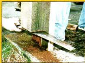
Rotted & infested base of a loadbearing column is completely sawed off and replaced with WoodEpoxy .
