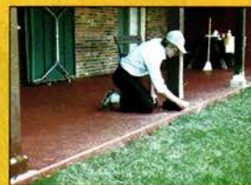
Rotted & infested base of a loadbearing column is completely sawed off and replaced with WoodEpoxy .
