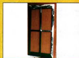
Antique window sash is salvaged, consolidated with LiquidWood and rebuilt with WoodEpoxy .
