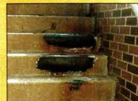
AboWeld 55-1, is much stronger than concrete and shapes without forms on steps and difficult surfaces.
