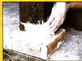
Rotted & infested base of a loadbearing column is completely sawed off and replaced with WoodEpox .
