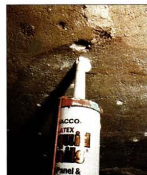
Left: Peter Lord prefers a commercial-size gun for reattaching the savable edges of this ceiling. Above: The \frac{1}{4} " injection hole is an effective size for a good seal with the adhesive tube.
