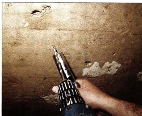
Top: Stained cracks and suspicious shadows—the telltale signs of a delaminating plaster ceiling. Above: Holding a vacuum nozzle on the drill bit helps suck the \frac{1}{4} " injection holes clear of dust.
