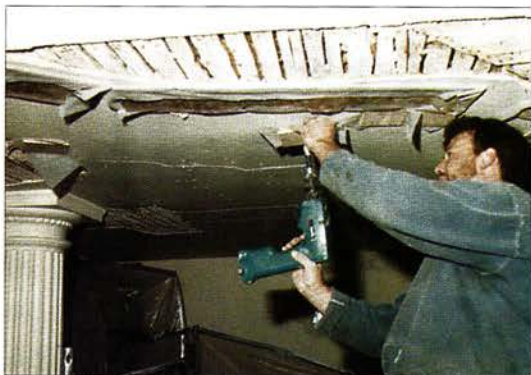
Top: Floor to ceiling shores hold the poly-coated forms in place. Note the pre-1840s split lath in the ceiling, and the industrial wet/dry vacuum in the background. Above: Screwing forms to the lath eliminates shores but adds holes.
