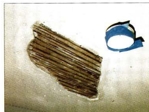
Top: Bulges too gone to reattach are best removed, then replastered. Above: Adding wire lath over wood lath improves an infill repair. Below: Like all good restoration, a successful repair is hard to see.
