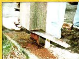
Rotted & infested base of a loadbearing column is completely sawed off and replaced with WoodEpox .
