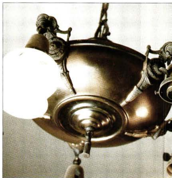
Examine light fixtures closely before making assumptions about metal finishes or polishing. What looks to be solid metal may actually be thin plating or even lacquer; the appearance of tarnish is sometimes an intended "antique metal" effect.
