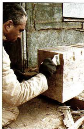
After the lintel is shaped, the crew seals the ends with melted wax so the oak dries slowly and with a minimum of checks and splits.
