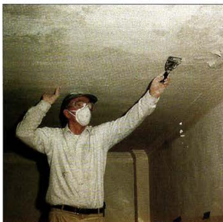
Above: Scraping off the failing paint is the first tedious step for dealing with calcimine problems. Oil-based paint dries to a firm, stiff finish, and will likely chip and flake away in small, crunchy pieces. Latex paint dries to a flexible, elastic finish, with a stretchy surface tension that causes it to peel away much faster and in large, rubbery pieces. Right: Carbide scrapers are handy for removing stubborn paint and even the calcimine itself.
