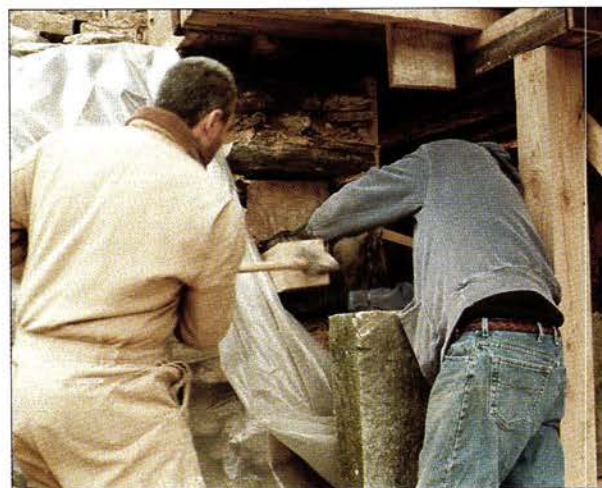
Top: Inside the basement, the crew slides the new lintel in place over the hearth using levers and muscle. Left: Outdoors, a swing with a sledhammer sets the lintel in place. Above: The end in its new home.
