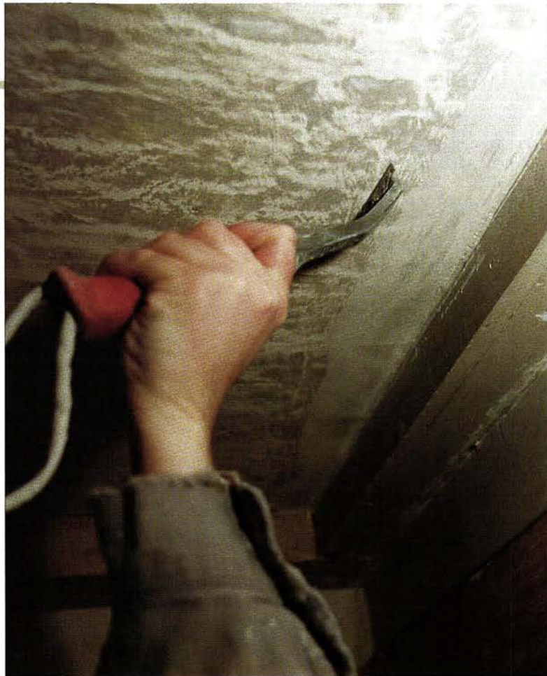
Above: Scraping off the failing paint is the first tedious step for dealing with calcimine problems. Oil-based paint dries to a firm, stiff finish, and will likely chip and flake away in small, crunchy pieces. Latex paint dries to a flexible, elastic finish, with a stretchy surface tension that causes it to peel away much faster and in large, rubbery pieces. Right: Carbide scrapers are handy for removing stubborn paint and even the calcimine itself.
