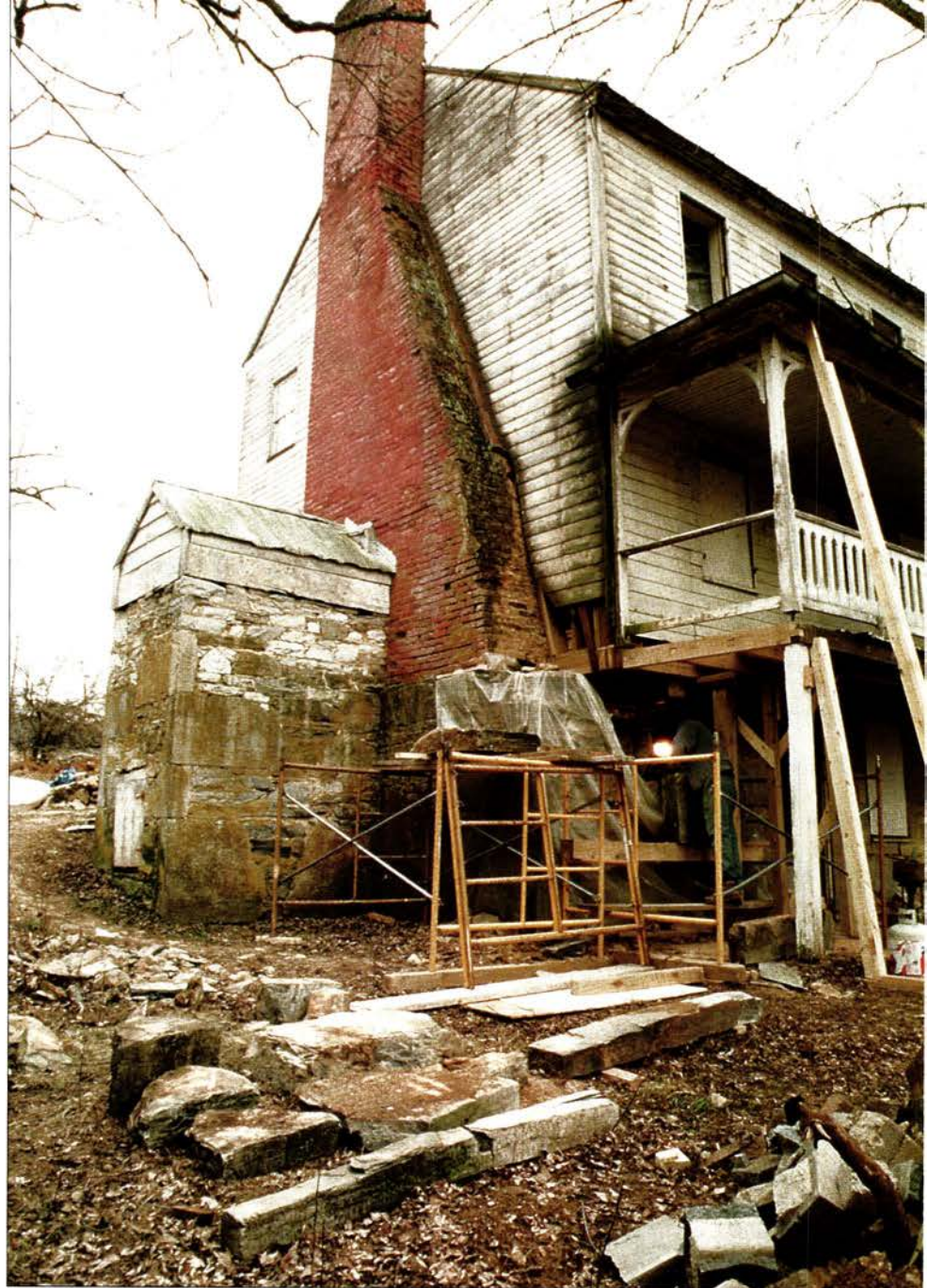
Above: The crew carefully dismantles part of the cooking hearth for later rebuilding. Each stone is carefully numbered and laid out in order of assembly.
