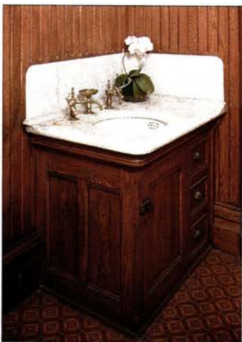
Fuller ball valves (above) were always lever handled. They appear in plain brass on this Victorian closed-plumbing lavatory (left).
