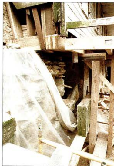
Above: The crew carefully dismantles part of the cooking hearth for later rebuilding. Each stone is carefully numbered and laid out in order of assembly.
