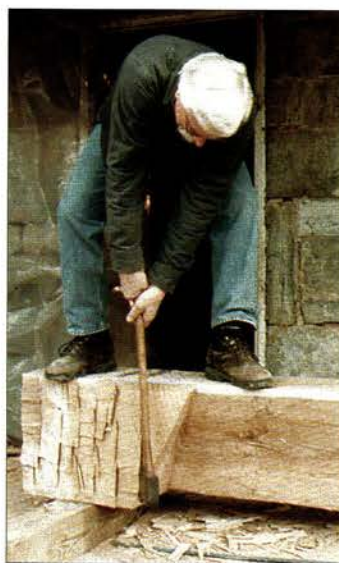
Next, standing on top of the timber, Doug swiftly scores the oak every 4" using the felling axe. Each kerf cuts no deeper than the chalk line dimension.
