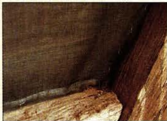
Screening will hold the Air Krete in place with 3" of clearance until it solidifies.
