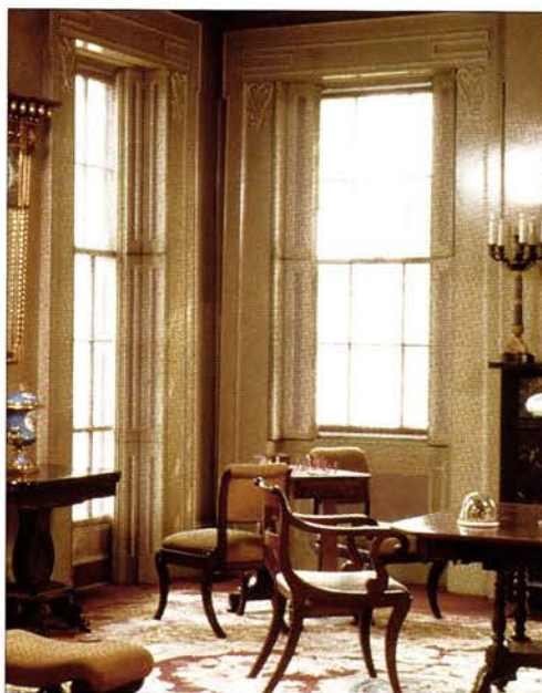
Thick-walled houses may have foldaway interior shutters, which can be quickly closed when sunlight is most direct and damaging.
