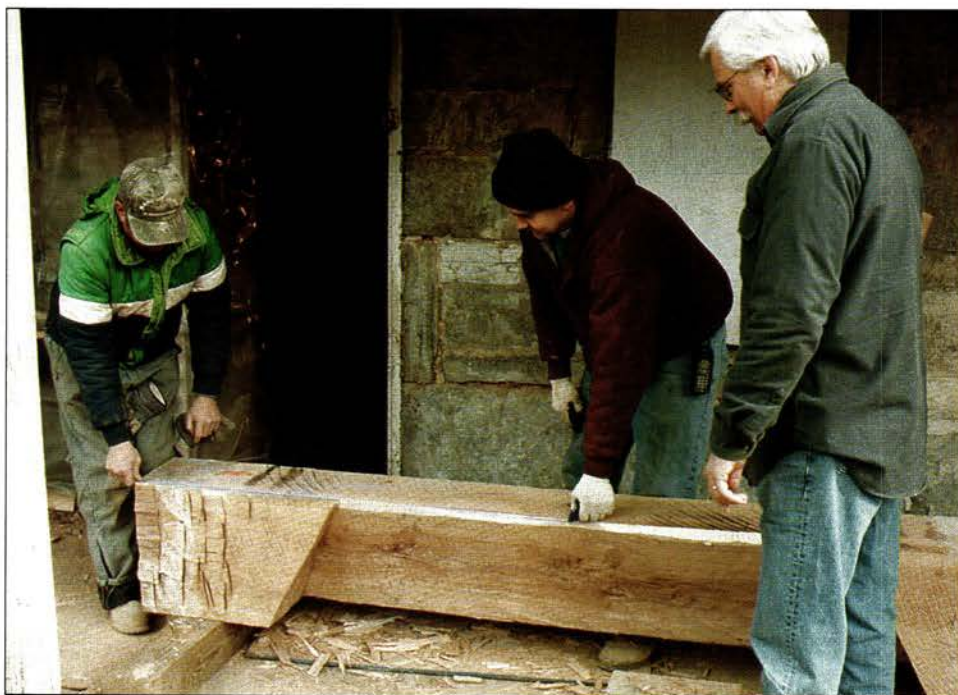
The first step in hewing one end of the massive lintel—some 600 pounds of green oak—is to snap a blue chalk line across the top to establish the new dimension.
