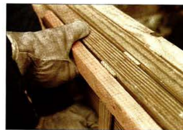
Left: Front porch framing replicates the mortised-and-tenoned oak framing. Above: On the back porch, the crew separates joists and trim boards with strips to promote breathing.
