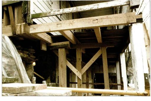
ers", hewn flat on one or two sides, then set with one flat side facing up. These sturdy members acted as flooring joists, and many survive to the present day. However, the outer edges of log joists have usually rotted away. Many later porches used simple frames constructed with 2x8 mill-sawn lumber to support the flooring. Unfortunately, these small-dimensioned frames are very susceptible to the water ever present on porches, which saturates the end-grain and quickly promotes rot.
