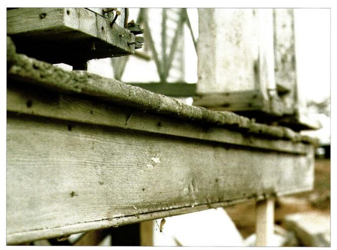
Left: These 150-year-old flooring boards are still intact because of their thickness and half-round bullnose edge, which provides more surface area for the ends to dry faster. Below: Back-cutting the decorative bandboards prevents water from accumulating behind the framing. Bottom: Though neglected, this 1850s porch is still standing because it is built with details that limit water intrusion.
