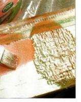
Citristrip (left), begins to work on the paint system immediately, after one thin application. Lead-X 40 (below) employees a lead immobilizer to change lead from a soluble to an insoluble-rendering the lead paint waste nonhazardous.
