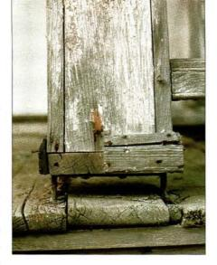
Early porch post feet (left) were simply iron bars bent into a stirrup shape. Manufactured versions (below) were common by the 1890s.
