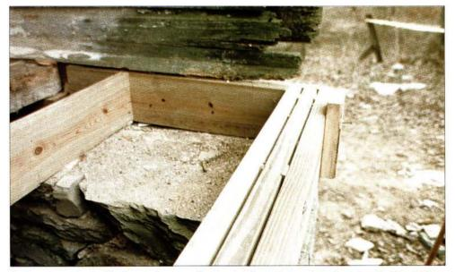
Modern pressure-treated lumber can be appropriate for rebuilding period porch framing where it will be hidden from view. In concealed locations, however, spacers between boards are even more important. Note that the shims are pressure-treated lumber as well.
