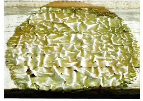
Soy-Gel, a biodegradable stripper made of soy ester and NMP, creates this "tenting" effect, separating the paint from the wood surface. The paint is then removed with a nonmetallic scraper.
