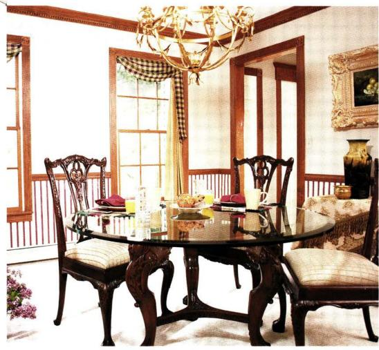
across its sharp lines to add detail and interest. It defines windows and doors within an elegant frame and anchors wall to floor with the baseboard. A shapely crown eases the transition from wall to ceiling, and a simple chair rail creates proportion. In the project shown here, a dining room needed a style upgrade that only new molding could create. Around the windows, plain clamshell molding was replaced by fluted casing, highlighted at the corners with rosettes. The passageway got the same
