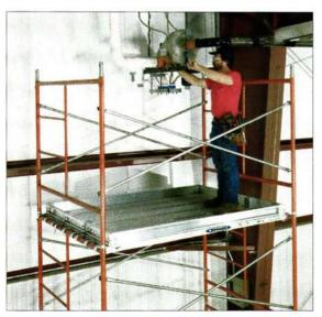
As you assemble a scaffold, remember to keep the rungs on each frame (far left in photo) positioned on the same side so that they make a continuous ladder.
