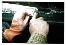
You can repair severely damaged wood, with deep gouges or even missing chunks, by filling it with epoxy fillers.
