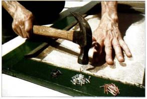
To rescreen, tack the mesh working from the middle of each side. Though bronze tacks can be hard to find, stick to the same metal as the mesh to avoid galvanic corrosion.
