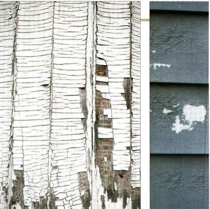
Above Left: Aptly named alligatored paint is usually the result of excess paint, all of which will have to be removed. Above Right: This paint is failing between coats, because of poor preparation or incompatible paint types or brands.
