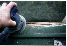
A sander is an essential tool for paint preparation, not only to help remove old paint coats but also to correct surface imperfections.
