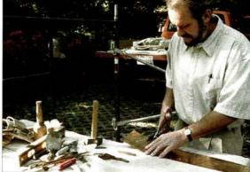
Above: Strike the setting mortar with a specialized tool to form the ropelike torus profile, keeping the horizontal bed joints continuous. Left: It's easy to make a joint-strike tool to reproduce a historic torus using copper flashing and common hand tools.
