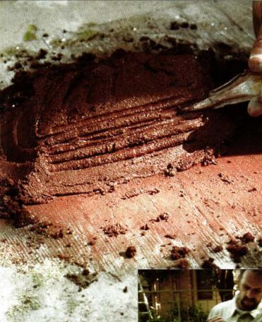
Above: Perfect your torus-making technique by working the strike tool in a test batch of stiff mortar: then adjust tool or mortar mix if necessary. Right: When repointing small areas, it's practical to simply mix mortar on the mortar board adding cements and pigments.
