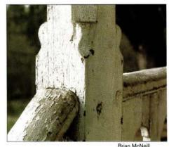
Above: It's easy to see the wood pins that still hold the tenons of these handrails snugly in the post mortises after 150 years.
