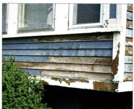
Above: What looks like dirt is often mildew, which will grow through new paint if not killed. Left: Paint peeling down to bare wood often signals excess moisture, from leaks or paint coats forming a barrier to vapor.
