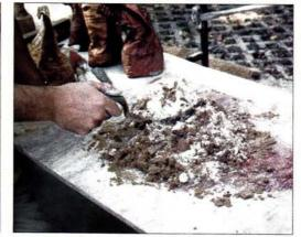
Small batches of mortar are convenient to mix on the mortarboard right next to your work. To ensure consistent color, thoroughly combine all dry ingredientscement, lime, sand, and pigment-before adding water. Keep track of proportions and measurements so that you maintain consistent mortar qualities from batch to batch.
