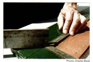
Thin screen bead mouldings (sold at good lumberyards) cover the tacks. Make quick miters by placing one bead over another (supported by scrap), then saw through both strips at once.
