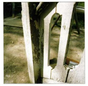
selected for durability, rather than mass-produced lumber shipped from a distant mill. It is this combination of thoughtful construction and the most durable materials that has kept many an early 19thcentury porch intact for 150 years. Using these details and materials, plus some newer ideas to augment the longevity of today's lumber, is the way we obtain the maximum life for porches.
