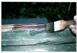
If wood is spongy or riddled with splitting, brush on a consolidant to strengthen it and bond epoxy fillers.
