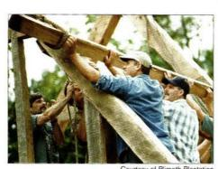
Courtesy of Plimoth Plantation The purlins are placed in the roof frame with wooden pegs.
