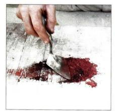
To mix colors, experiment with pigment and remember that in the first week the mortar will look darker than the final cured color. To produce brown, mix black and red mortar pigments; for buff, mix white, yellow, and red; for straw color, yellow and white; for orange, yellow and red.
