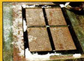
Antique window sash consolidated with LiquidWood and rebuilt with WoodEpoxy .
