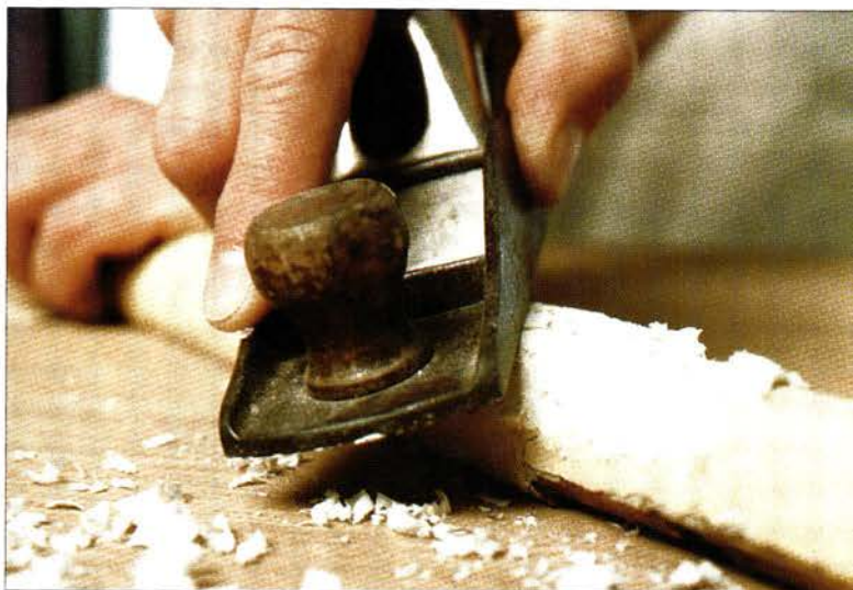
Above: When cured, epoxy fillers formulated for wood restoration can be shaped and sanded the same as hardwoods. Below: Fillers are also effective for reconstructing the lost portions of complex decorative elements, such as this football-sized newel cap. The deterioration at the core is typical of conditions that require drying and perforating the wood before consolidating. Bottom: In advanced applications, epoxies are also used to rebuild beams. In this model, horizontal fiberglass rods reinforce an epoxy prosthesis cast in place on a rotten beam end.
