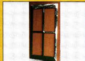
Antique window sash consolidated with LiquidWood and rebuilt with WoodEpoxy .
