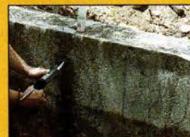
AboJet for structural crack-injection
