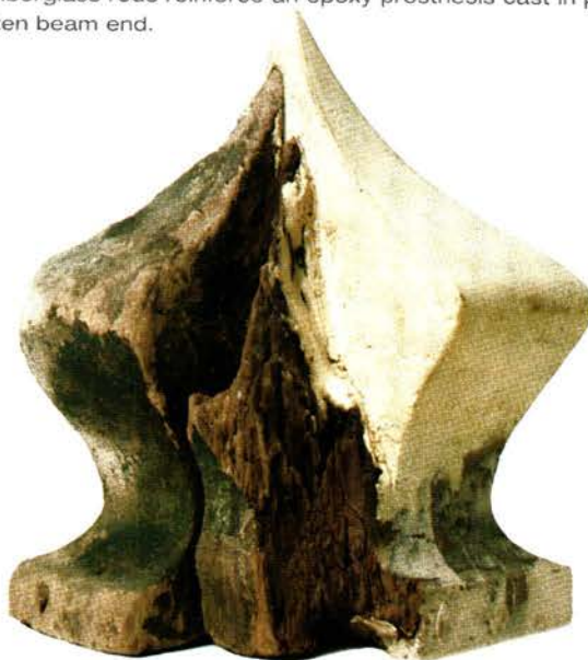
Above: When cured, epoxy fillers formulated for wood restoration can be shaped and sanded the same as hardwoods. Below: Fillers are also effective for reconstructing the lost portions of complex decorative elements, such as this football-sized newel cap. The deterioration at the core is typical of conditions that require drying and perforating the wood before consolidating. Bottom: In advanced applications, epoxies are also used to rebuild beams. In this model, horizontal fiberglass rods reinforce an epoxy prosthesis cast in place on a rotten beam end.
