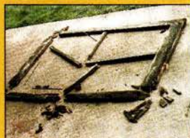
Antique window sash consolidated with LiquidWood and rebuilt with WoodEpoxy .
