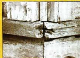
Consolidation and rebuilding of rotten windowsill with LiquidWood and WoodExpo .
