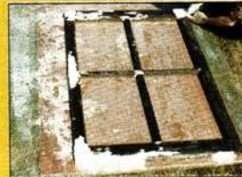
Antique window sash consolidated with LiquidWood and rebuilt with WoodExpo .
