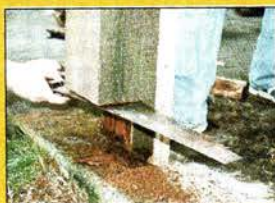
Rotted loadbearing column base sawed off and replaced with WoodExpo .
