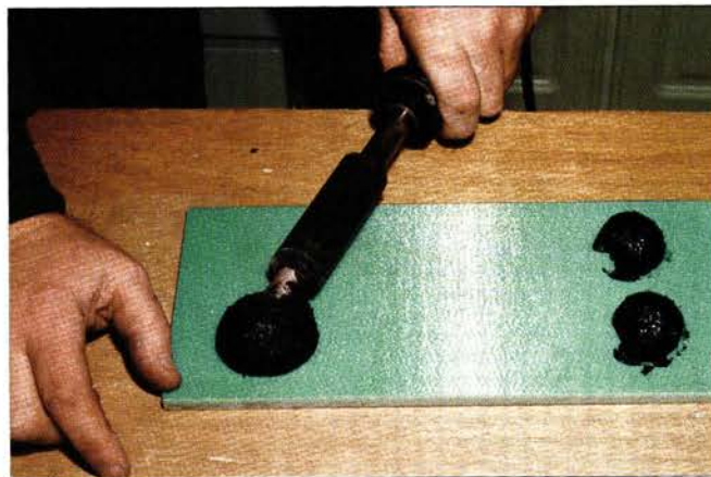
Vitrolite is scored for cutting (left), similar to ceramic tile or window glass. Dunn then applies mastic with an electrically heated scoop applicator (right) before installing the tile on the primed wall (below right).
