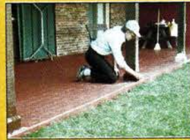
Rotted loadbearing column base sawed off and replaced with WoodExpo .
