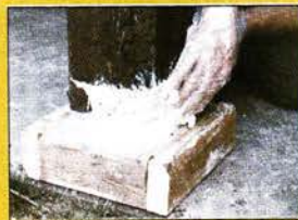
Rotted loadbearing column base sawed off and replaced with WoodExpo .
