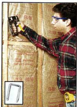
Install Insulation
