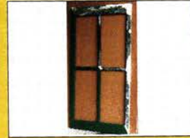
Antique window sash consolidated with LiquidWood and rebuilt with WoodExpo .
