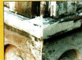
Consolidation and rebuilding of rotten windowsill with LiquidWood and WoodExpo .
