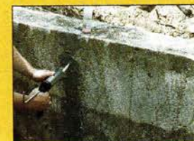
AboJet for structural crack-injection
