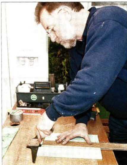
Vitrolite is scored for cutting (left), similar to ceramic tile or window glass. Dunn then applies mastic with an electrically heated scoop applicator (right) before installing the tile on the primed wall (below right).
