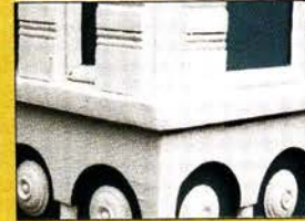
Consolidation and rebuilding of rotten windowsill with LiquidWood and WoodExpo .
