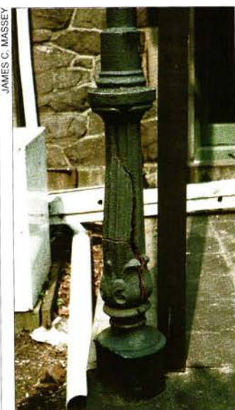
Top: Check window and balcony railings for rust where they meet the building, a condition that can indicate failing ironwork. Above: Damaged structural cast iron should be replaced, not repaired.
