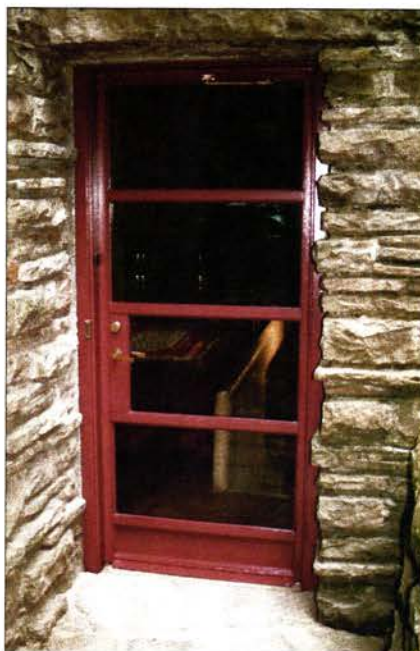
Left: The Conservancy feared that the bridge entrance (in effect, a large steel window) would have to be replaced, but patching allowed the crew to retain nearly all the original parts. Below: Bob Seekircher brazes replacement steel into the door frame.
