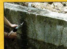
AboJet for structural crack-injection
