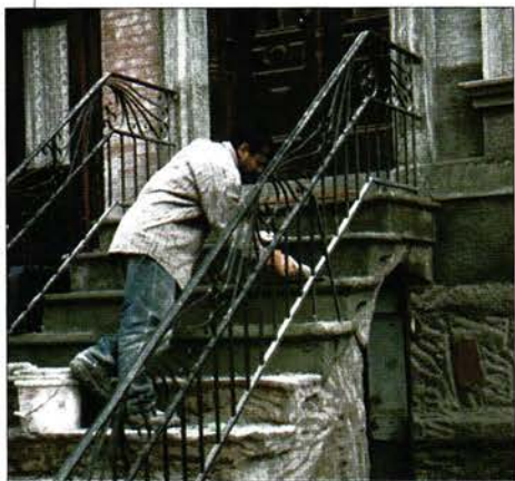
A mason applies patching material to the front steps of the Fort Green brownstone. Note the scratch marks in the stone.
