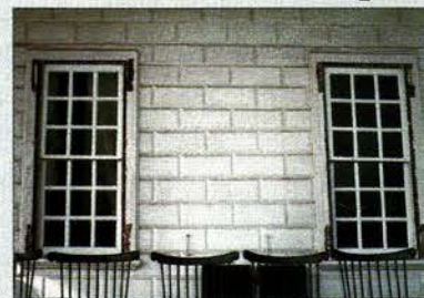
Stripping the parlor window casings on the mansion's east-side revealed clues to the original hinge style.
