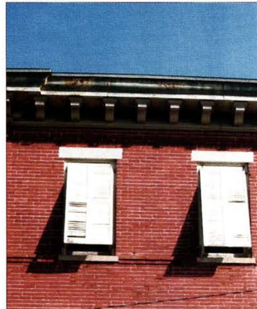
Do's: These paneled shutters (above left) and the board-and-batten reproduction shutters from Timberlane Woodcrafters (top) swing on pintle hinges and sport shutter dogs to hold them open. Awning or Bermuda hinges (above) are popular in the subtropics where they block sun while letting in breezes. For more information on Timberlane, circle 30 on resource card.
