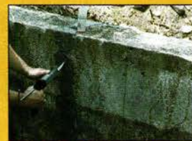
AboJet for structural crack-injection
