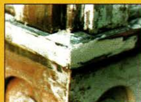
Consolidation and rebuilding of rotten windowsill with LiquidWood and WoodEpox .
