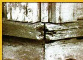
Consolidation and rebuilding of rotten windowsill with LiquidWood and WoodEpox .
