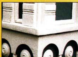
Consolidation and rebuilding of rotten windowsill with LiquidWood and WoodEpox .
