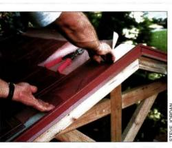
The next shingle is installed by sliding it into place on the previous shingle so that they interlock. This basic process is repeated across the roof and up, course by course.
