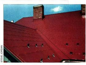
Typical of many old houses, completing the Grieve roof required flashing at valleys and intersecting gable ridges in matching materials supplied by the shingle manufacturer.
