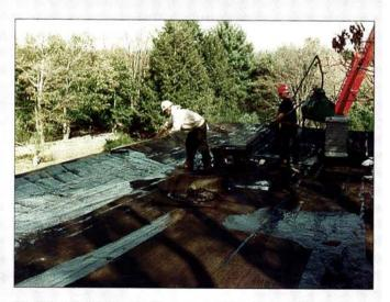
The flat roof at the Gropius House presented another set of leakage problems, some precipitated by the gravel stop flashing. Originally the gravel stop along the roof edge was a continuous piece of flashing that joined the built-up roof in a lapped and flood-coated joint (top drawing). Years of thermal expansion broke this seam. Our solution was to add periodic expansion joints along the length of the flashing, and to bring the roof up to it over a tapered edge strip.
