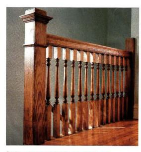
Stairs came completely manufactured and ready to nail in place. Every part of the stairs—newels, balusters, railing, risers, treads, and stringers—was keyed by number for easy assembly.
