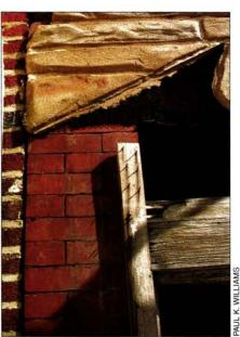
your crowbar to avoid chipping into the brick or wood. On brick surfaces focus on nail points in the lath, usually placed in the mortar joints. In most cases the weight of the simulated masonry will break the lath or chicken wire; if not, you may need the wire cutters.
