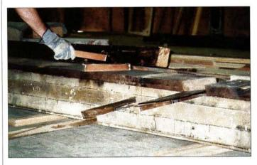
approximately 350 pounds. In order to join the two timbers, the original carpenter hadn't used nails or bolts, but a simple and elegant system that relied on strategic cutting to essentially forge one joist out of two. This technique, described in the accompanying photos, is a variation of the scarf joint, a staple of 19th-century heavy carpentry.
