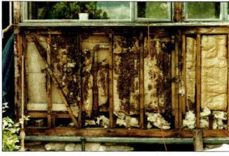
Coming from the windows, water bypassed the major waterproofing element in the walls—the asphaltic felt to deteriorate the framing and other materials behind it. Note the decaying studs and batts of Cabots Quilt, an early thermal insulation product made with eel grass (a kind of sea grass).
