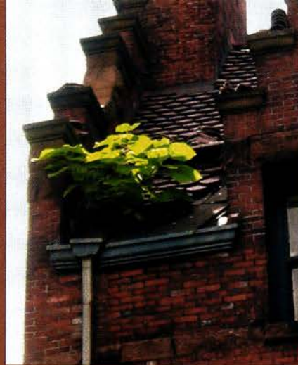
Plants in any gutter can grow quickly, with roots (or stems in the case of ivy) loosening tiles and causing them to crack or break.
