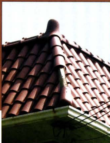
A missing ridge tile invites water or ice to penetrate under the remaining roof tiles below it.
