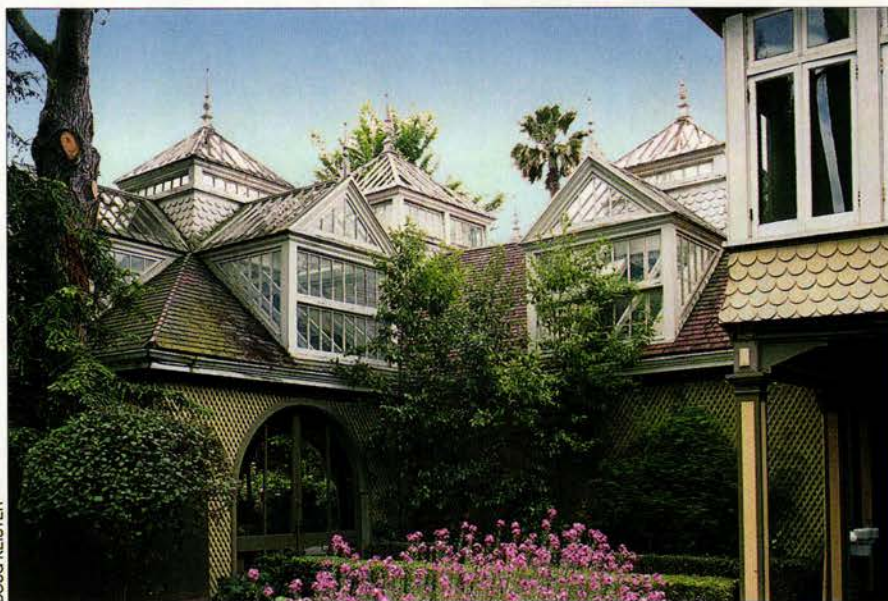
Above: At the Winchester House in San Jose, California, a series of skylight dormers and roof lanterns set into a solid roof shelter the greenhouse below.
