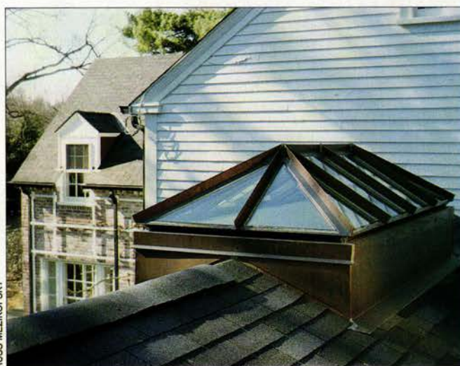
This copper, hipped skylight designed by Peter Hosmer of Charles River Restoration is a reproduction from a late 19th-century model. Note the skylight's curb.
