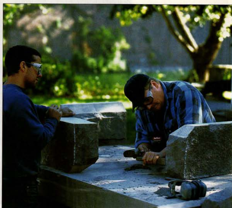
Mark Favale watches while Rick Lane dresses stone. While much heavy quarrying and stone shaping is mechanized, detailing is still a traditional, hand process.
