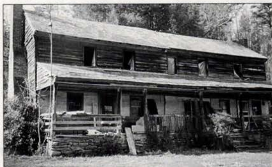
Rotten sills had caused the house, unoccupied for two decades, to sink toward its center.
