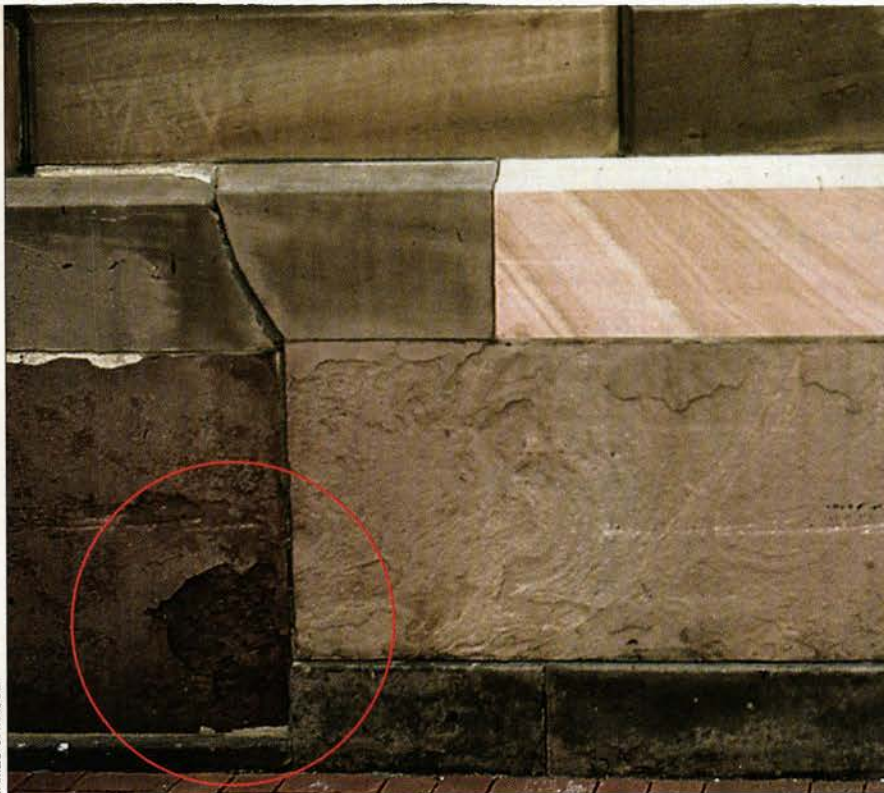
The scourge of brownstone buildings is flaking of the stone along the sedimentary layers (in circle), a failure usually precipitated by face-bedding blocks with their layers vertical. In-kind stone replacement (light stone) is a more satisfying repair.
