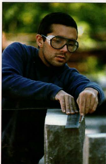
Making the rock face that decorates most ashlar (rectangular) brownstone begins by establishing the edge.
