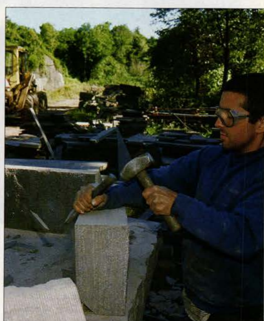
Controlled spalling of the stone edge with a hammer and chisel creates this traditional detailing.
