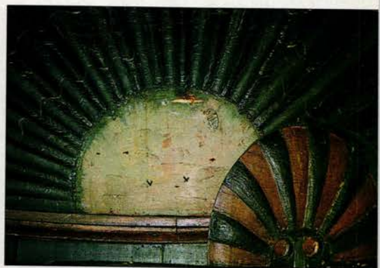
Close inspection of the shell cupboard paint showed carving highlights picked out in brown. Under a lens, however, this "paint" proved to be the bonding agent for gold leaf that had long since disappeared.
