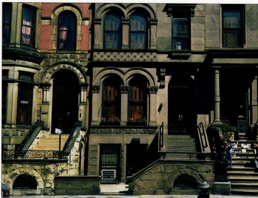
Romantic in color and readily carved, brownstone was the fad facing for Italianate-style row houses of the late 19th century—especially in New York City, where the ubiquitous buildings are known as brownstones. By 1900, however, the stone was decidedly passé.
