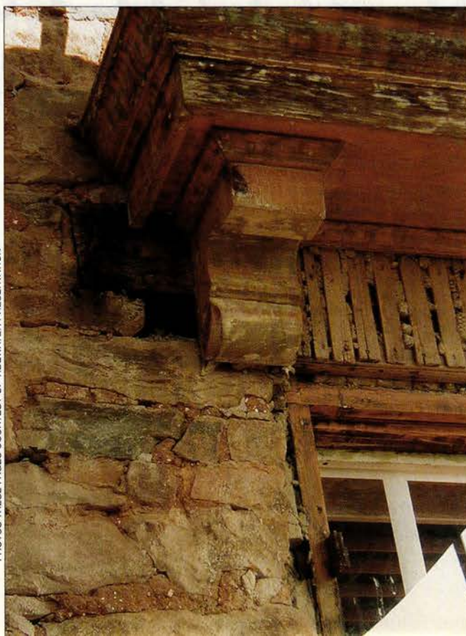
The crew removed the stucco using crowbars. Once the stucco was off, the underlying wood around doors and windows showed signs of rot and had to be replaced.
