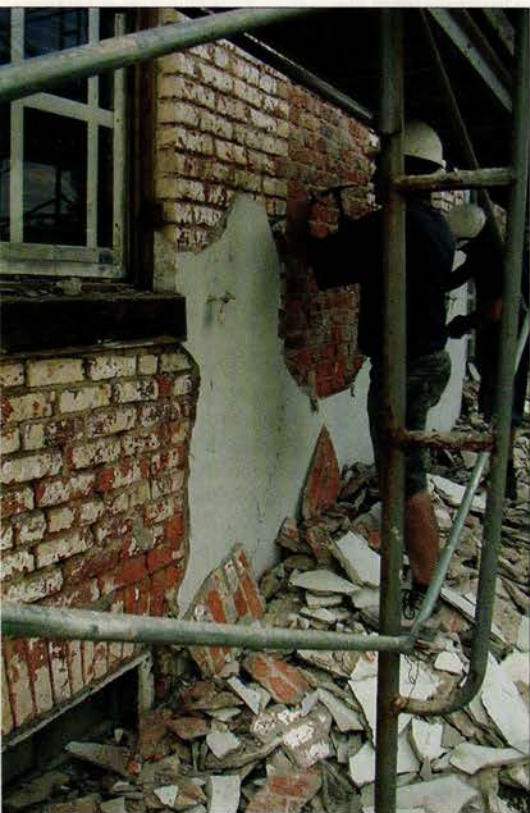
The crew removed the stucco using crowbars. Once the stucco was off, the underlying wood around doors and windows showed signs of rot and had to be replaced.
