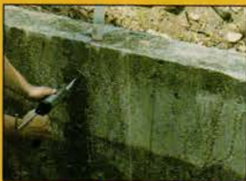
AboJet for structural crack-injection
