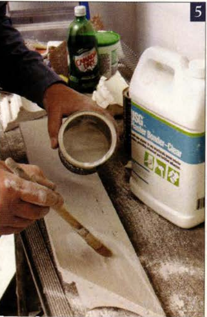
Left: After test fitting and roughing up the back of the patch, Peter brushes on bonding agent to aid adhesion.
