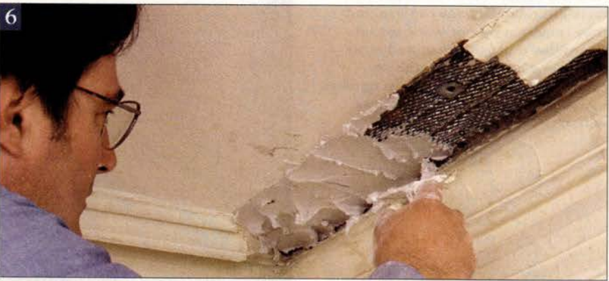
Left: After test fitting and roughing up the back of the patch, Peter brushes on bonding agent to aid adhesion.
