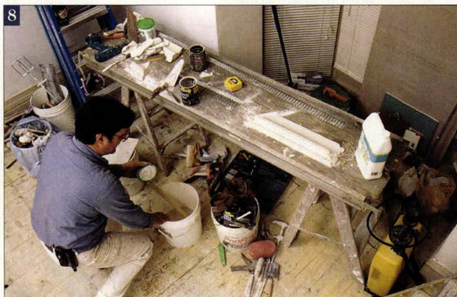
Above: Plaster repair materials and tools are relatively easy to use, but they require a proper work set up. Quantities must be measured accurately, and containers and tools cleaned scrupulously between batches to avoid contaminating a new mix with bits of hardening plaster.
