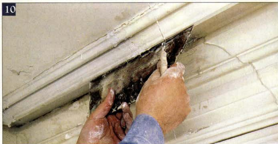
Peter blends in the repair with a miter rod—a traditional tool used to shape corners and joints in cornice work. Drawing the tool down across the cornice, while it bridges new and old, forms the wet plaster along the joint.
