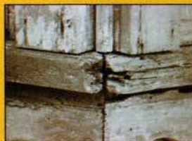
Consolidation and rebuilding of rotten windowsill with
