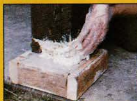
Rotted loadbearing column base sawed off and replaced
