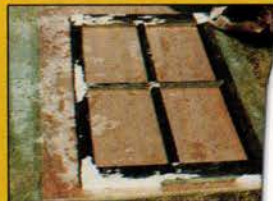
Antique window sash consolidated with LiquidWood and
