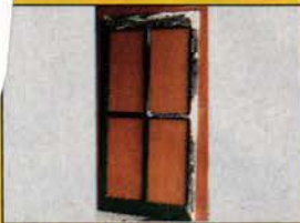
rebuilt with WoodEpox.
