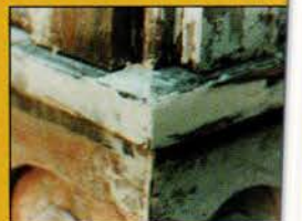
Consolidation and rebuilding of rotten windowsill with
