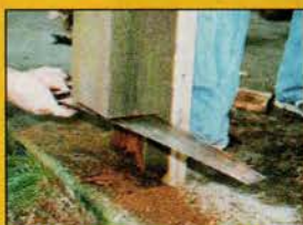
Rotted loadbearing column base sawed off and replaced
