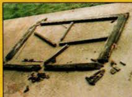
Antique window sash consolidated with LiquidWood and
