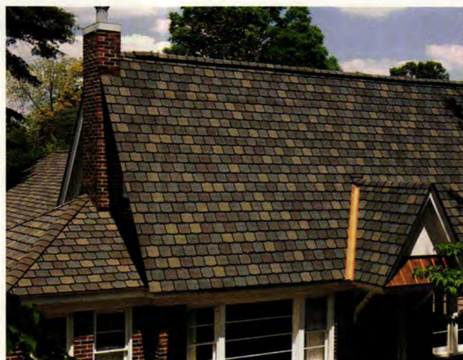
Above: Concrete tile, already close to architectural slate in thickness, bears a striking resemblance in products like Natural Slate from Vande Hey-Raleigh. Left: Manufacturing technology that varies color not only from tab-to-tab but across tabs adds another level of realism to slatelike asphalt shingles such as Centennial Slate from Certainteed.
