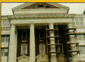
MasterMold makes molds of architectural elements in situ.
