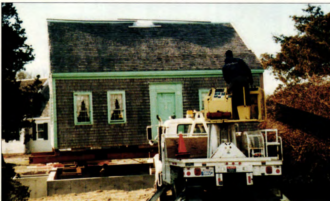
Once it reached its final destination, the house was placed onto its foundation.
