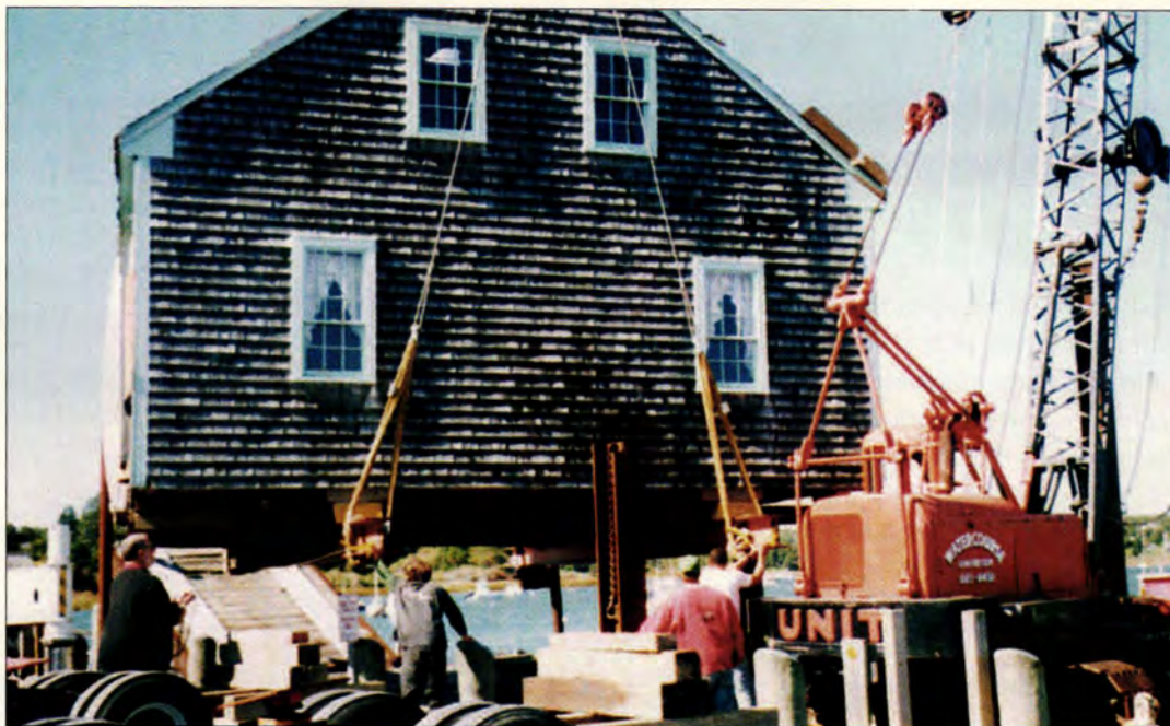
A crane with a heavy-duty spreader bar lifted the house and placed it on the barge.
