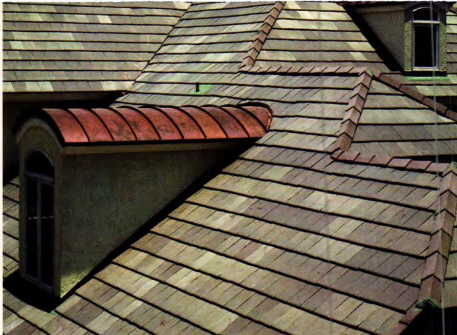
Above: Clay tile, shaped and glazed with naturalistic variations, has historic precedent as a slate imitator and is available today in products lighter than stone, such as Celadon Ceramic Slate. Left: Today's slate-like asphalt shingles, such as Capstone from Elk, also come in a wider range of historic slate colors beyond the basic greys and blacks.
