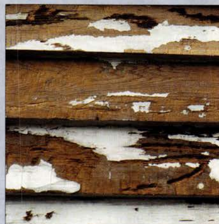
High-pressure streams from water blasting will penetrate paint and even eat gullies and holes in wood fiber.
