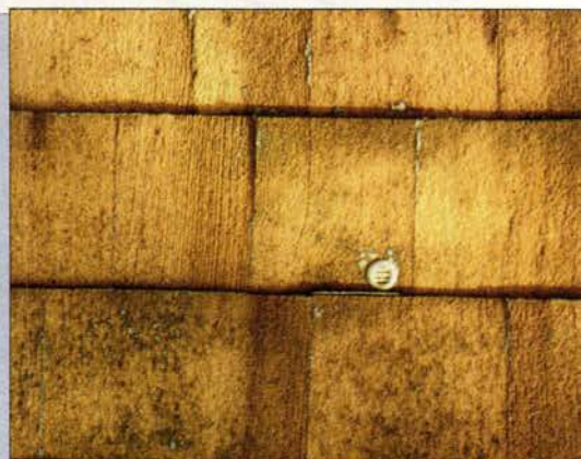
Never gentle on wood, sandblasting has eroded away the softest parts of these once-smooth cedar shingles.
