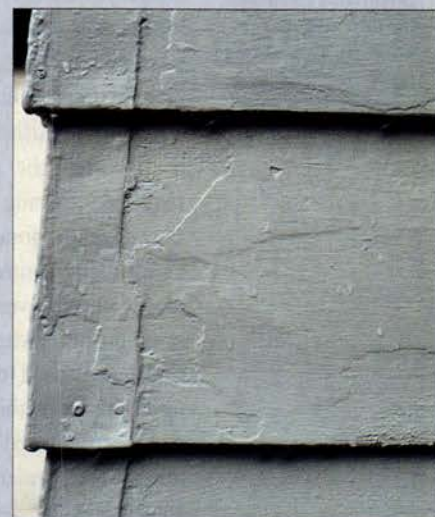
Unsightly craters are the sign of thick paint build-up that has peeled in places, then been scraped and repainted.
