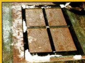
Antique window sash consolidated with LiquidWood and rebuilt with WoodEpox .
