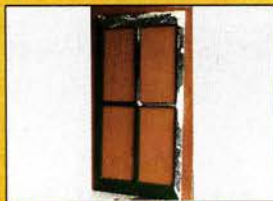
Antique window sash consolidated with LiquidWood and rebuilt with WoodEpox .
