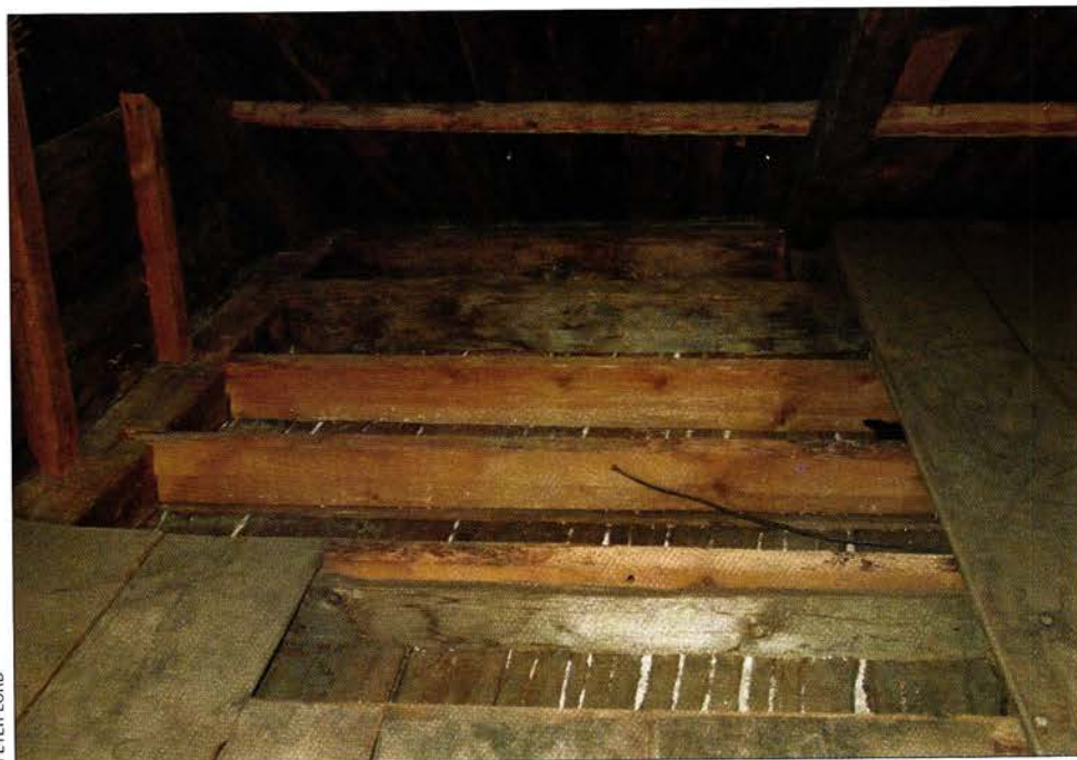
The dimensions of the bays (voids) between joists usually determine the amount of attic insulation, but it's possible to add more by raising the floor on furring.
