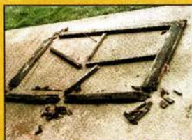
Antique window sash consolidated with LiquidWood and rebuilt with WoodEpox .
