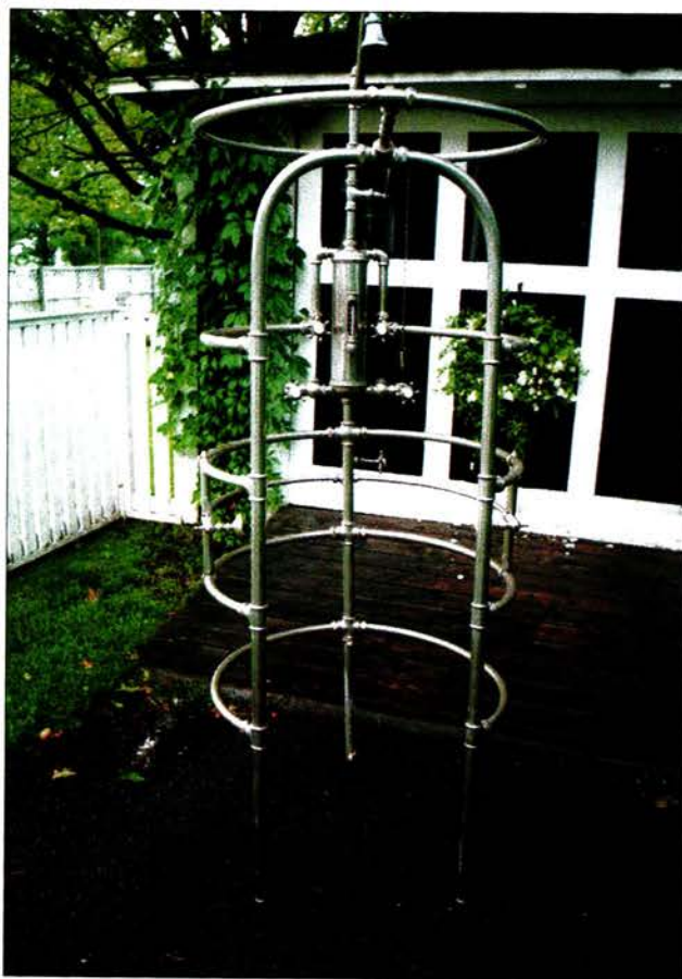
This 1922 cage shower from Hoffman & Billings of Milwaukee is typical of the kind made by a half-dozen manufacturers in the 1910s. Note the large mixing manifold at the back surrounded by valves to control the various showers.
