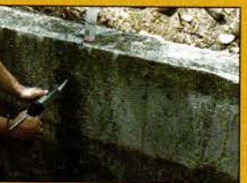
AboJet for structural crack-injection
