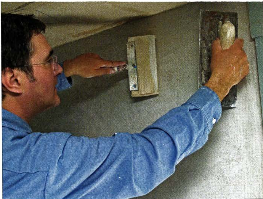
When the plaster has taken an initial set and is firm enough to work some more, Peter uses a felt ahead of his trowel to add moisture that keeps the surface workable to remove trowel wakes and achieve desired smoothness.
