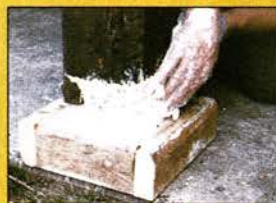
Rotted loadbearing column base sawed off and replaced with WoodEpox .
