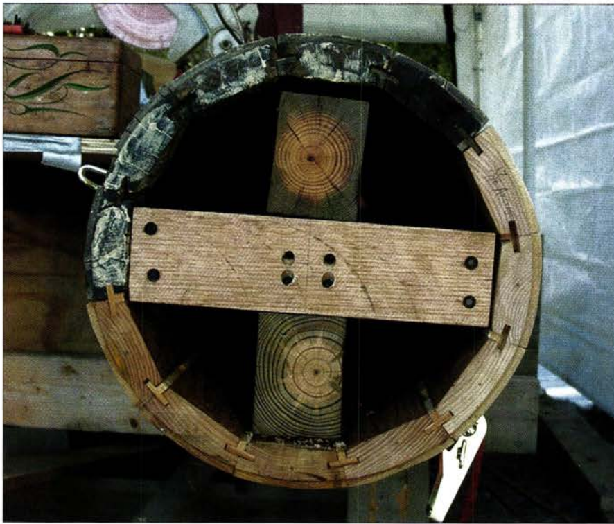
Beefing up the post system inside the column included adding two 4x4s as well as a second bar across the bottom to make an X platform.
