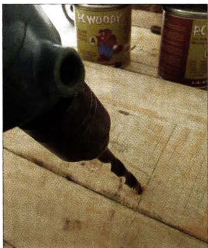
Severing each stave meant making a blind cut in the middle of the column, starting with a \frac{3}{8} " hole.
