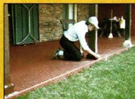
Rotted loadbearing column base sawed off and replaced with WoodEpox .
