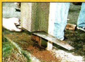
Rotted loadbearing column base sawed off and replaced with WoodEpox .
