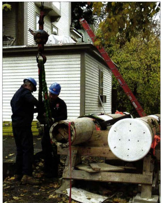
The columns, waiting for reinstallation, show a rebuilt bottom with vent holes, next to a top, still in good condition.
