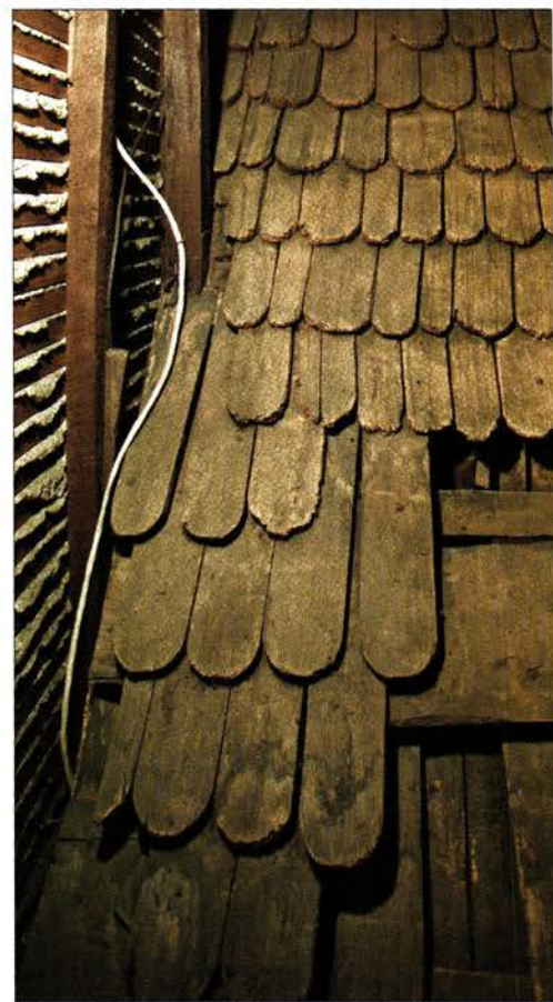
The 18th-century addition was built over the existing roof, preserving its wooden fishscale shingles, which can still be seen from an attic space on the second floor.
