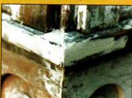
Consolidation and rebuilding of rotten windowsill with LiquidWood and WoodEpoxy .
