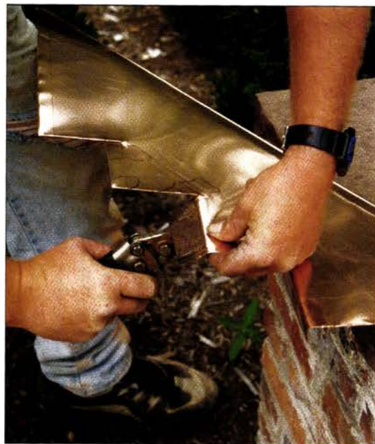
Most old-house chimneys (left) are made of porous brick or stone. In quality work, they are built with through-wall flashings to block moisture, and any new flashing (below) should be added so as to work with this system.
