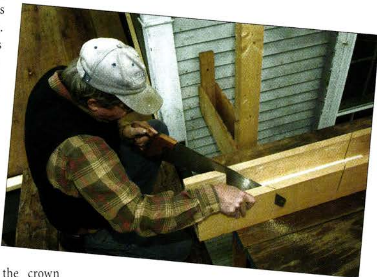
The cornice miter box (above) is custom-made to fit the height and projection of the crown moulding. Finessing the joint with a Japanese saw (below) brings the mouldings into a tight miter.
