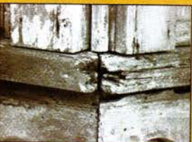
Consolidation and rebuilding of rotten windowsill with LiquidWood and WoodEpoxy .
