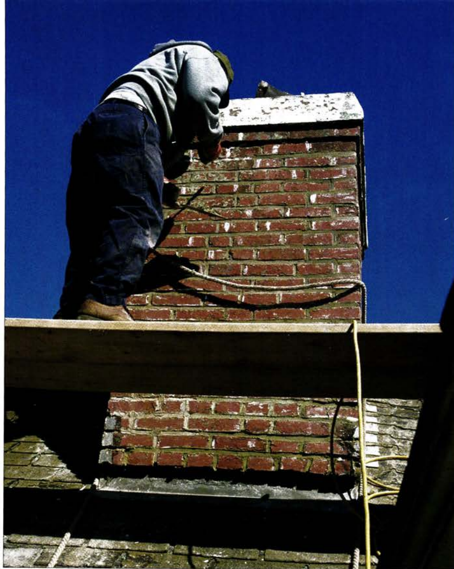
Most old-house chimneys (left) are made of porous brick or stone. In quality work, they are built with through-wall flashings to block moisture, and any new flashing (below) should be added so as to work with this system.
