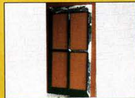
Antique window sash consolidated with LiquidWood and rebuilt with WoodExpo .
