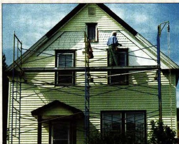
Removing the vinyl siding revealed wood shingles—surprisingly intact, but still due for repainting.
