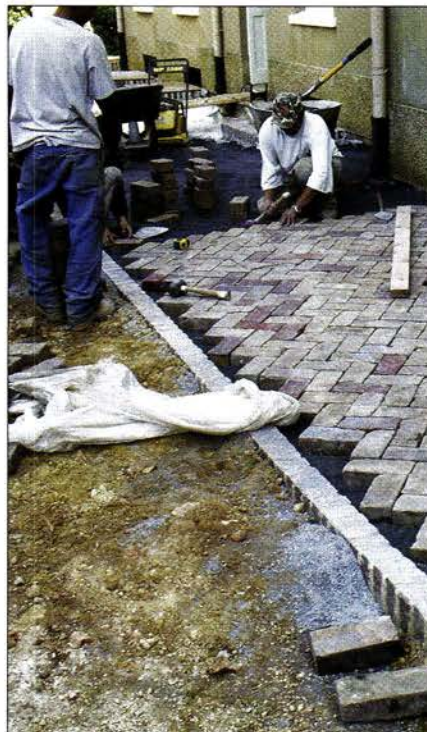
Masons carefully dry-laid bricks in a diagonal herringbone pattern using string lines to lay out leading corners.
