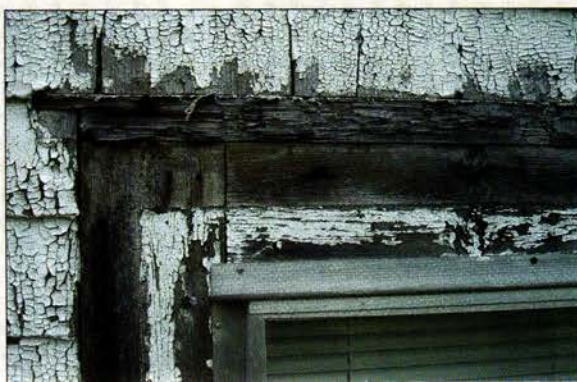
The siding installers' legacy included window sill ends cut back to the casings (above) and headers completely lost but for their paint ghosts (below).
