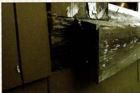
The siding installers' legacy included window sill ends cut back to the casings (above) and headers completely lost but for their paint ghosts (below).
