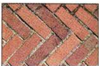
Herringbone: Bricks laid zig-zag at 45 degrees to row direction.
