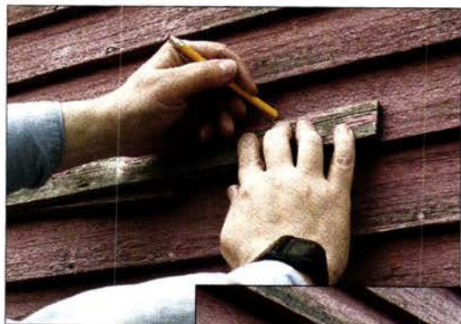
The first step is to cut the patch material, then lay it over the damage and trace the outline. Right: Next saw to the end lines with a cross-cut saw.
