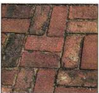
Basket weave: Groups of two or three bricks laid in alternating directions.
