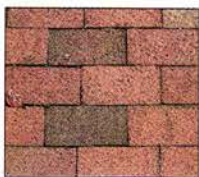
Running bond: Joints fall half- way between adjacent rows.
