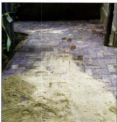
After carefully tapping bricks in place in dry stone dust (top left), sweeping masonry sand into joints (bottom left) adds vertical and horizontal support. The finished walkway (above) is a dead ringer for the 1914 version it replaced.
