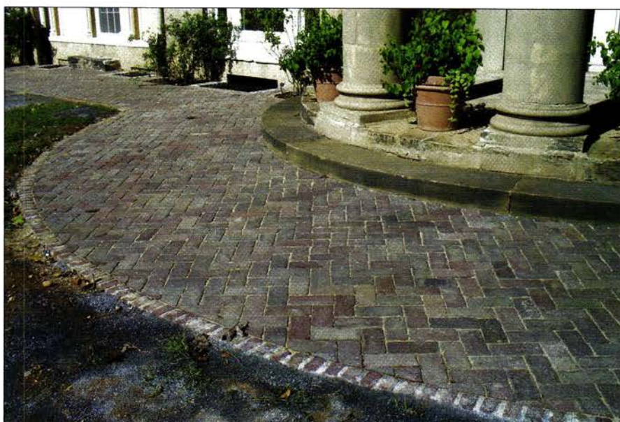
After carefully tapping bricks in place in dry stone dust (top left), sweeping masonry sand into joints (bottom left) adds vertical and horizontal support. The finished walkway (above) is a dead ringer for the 1914 version it replaced.
