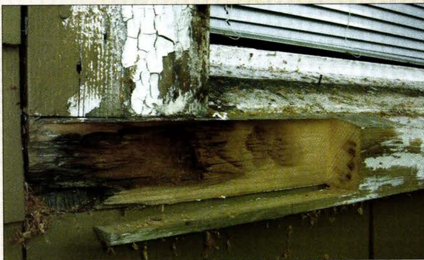
The challenge of the sill ends (above) was to create a joint that would minimize weather exposure while making a good mechanical connection. The solution was to rout the sill back under the casing (to cover much of the joint), and into the middle of the window a couple of inches at a bevel.
