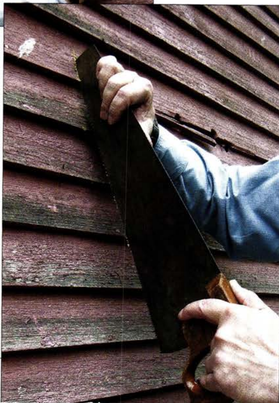
The first step is to cut the patch material, then lay it over the damage and trace the outline. Right: Next saw to the end lines with a cross-cut saw.
