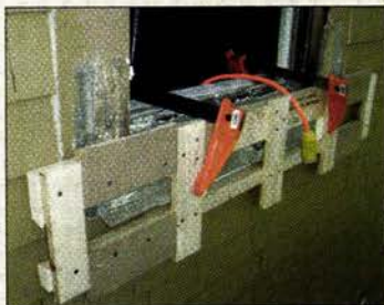
A jig built to fit all window sizes allowed the \frac{1}{2} " plunge router to cut back sill ends to uniform dimensions.
