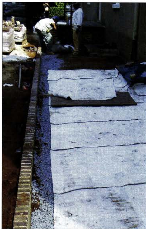
Layering bentonite fabric across the surface and extending it 1" over the drain added waterproofing.
