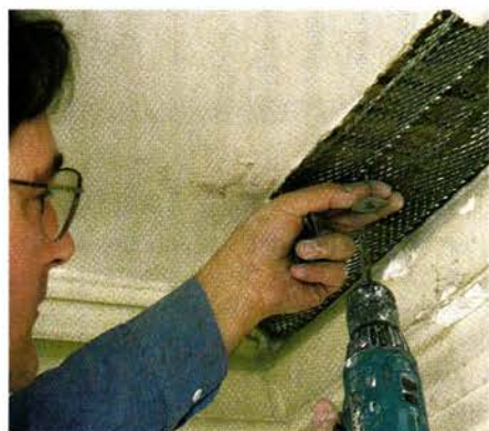
Expanded metal mesh is the modern lath common since the 1920s and widely used for large repairs. Here, a piece is cut to the patch shape and screwed right over the old wood lath to improve anchoring for the plaster scratch coat.
