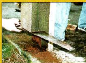
Rotted loadbearing column base sawed off and replaced with WoodEpoxy .
