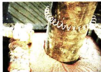
Like many retrofit liners, the new flue in cast-in-place liners is smaller in cross-sectional area than the old flue.
