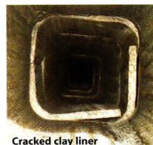
Cracked clay liner
