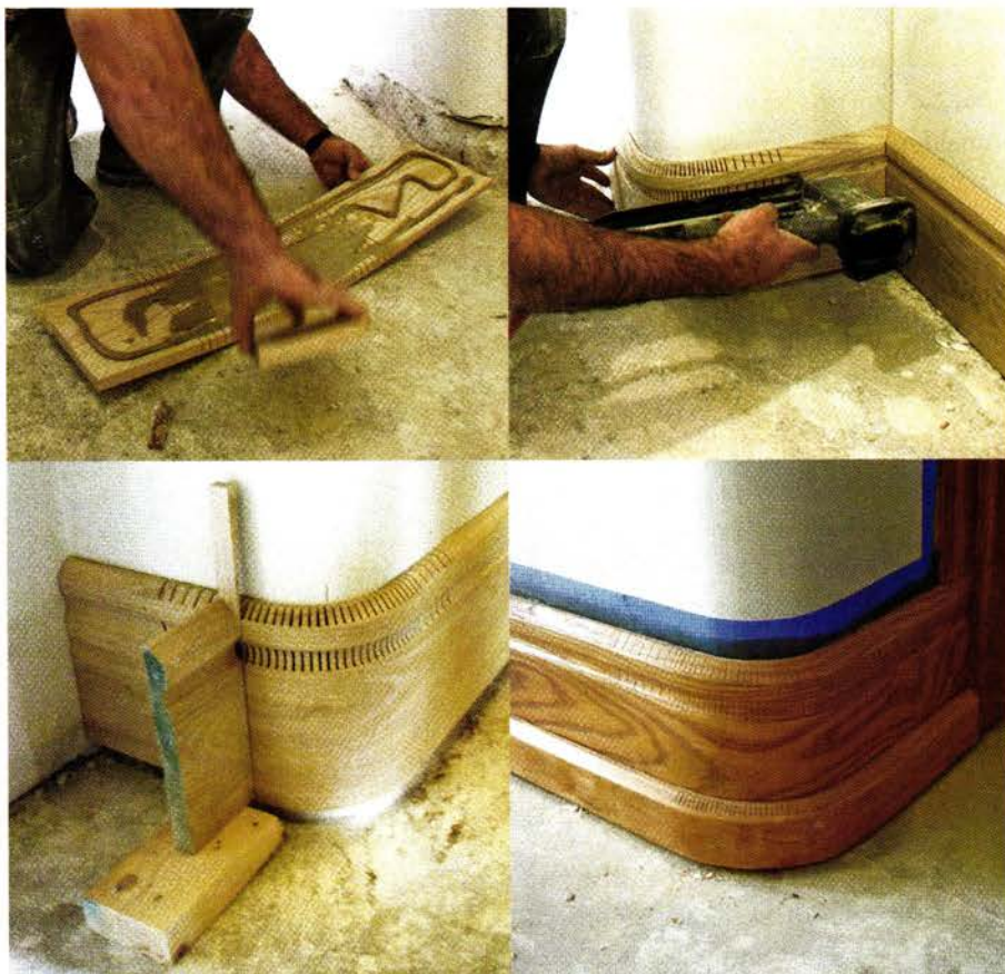
CLOCKWISE: At installation, boards are spread with glue, pinned into place using a pneumatic nail gun, and bolstered with a pressure block until the glue sets up. The finished baseboard, with the addition of stain and a similarly kerfed shoe moulding, looks just like the originals.
