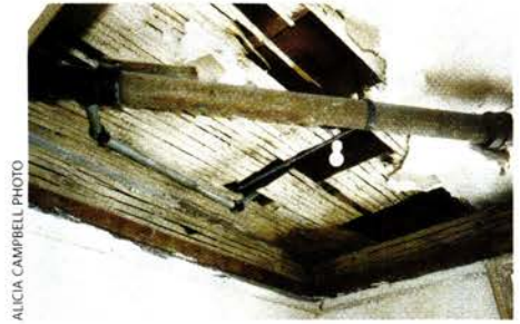
ABOVE: Getting rid of the downstairs bathroom's dropped ceiling exposed an enormous, cast iron waste pipe that ran diagonally across the room. While removing it, the couple learned the benefits a solid sense of humor provides. LEFT: The finished bath's period details belie its remuddled past.
