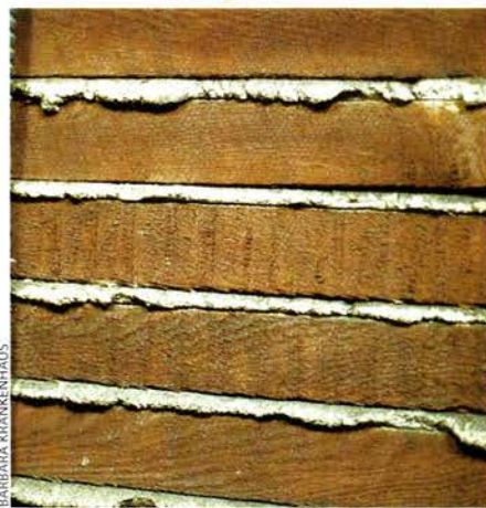
LEFT: When wet plaster penetrates the lath and hardens, it forms keys that are the mechanical anchors of the wall. When these keys break, the three coats of plaster will migrate away from the lath, but can sometimes be reattached if there is access to inject adhesive. RIGHT: Plaster washers may be practical for re-anchoring plaster where the only access is from the finish side.
