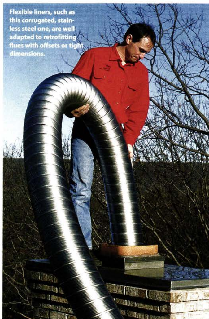
Many old-house chimneys serve a hearth on each floor with multiple flues that snake through offsets within the masonry.
