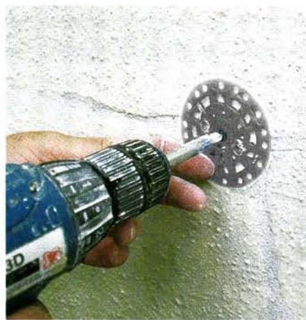
LEFT: When wet plaster penetrates the lath and hardens, it forms keys that are the mechanical anchors of the wall. When these keys break, the three coats of plaster will migrate away from the lath, but can sometimes be reattached if there is access to inject adhesive. RIGHT: Plaster washers may be practical for re-anchoring plaster where the only access is from the finish side.
