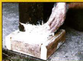
Rotted loadbearing column base sawed off and replaced with WoodEpoxy .
