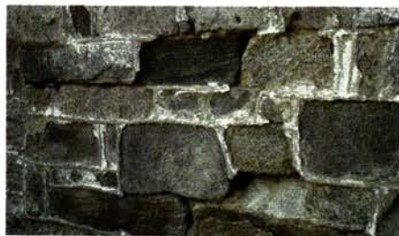
The results of too-hard mortar can be spalling of soft, pre-1860s brick (top) and some soft stones such as rubble fieldstones (bottom).
