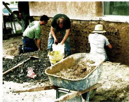
HCN workers use porous stone and adobe plaster to repair a home in Mesilla, New Mexico.
