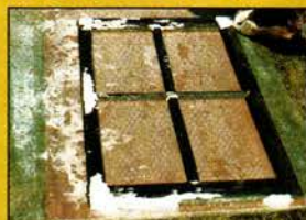
Antique window sash consolidated with LiquidWood and rebuilt with WoodEpox .
