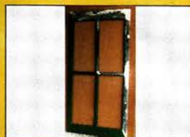
Antique window sash consolidated with LiquidWood and rebuilt with WoodEpox .
