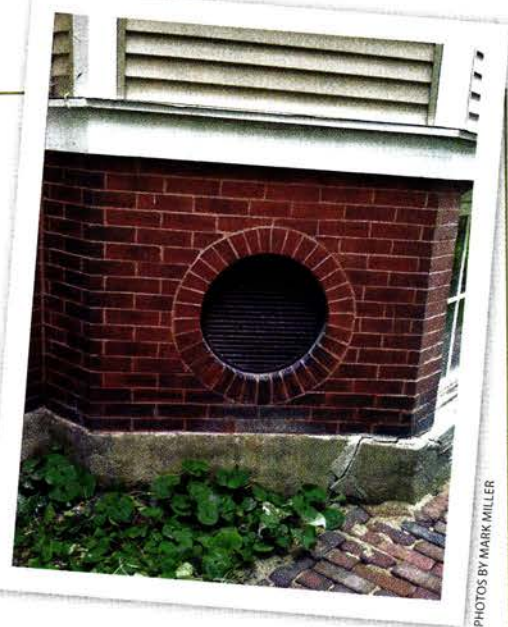
ABOVE: A round air grille appears about 3' above grade on a tony Victorian's exterior.
