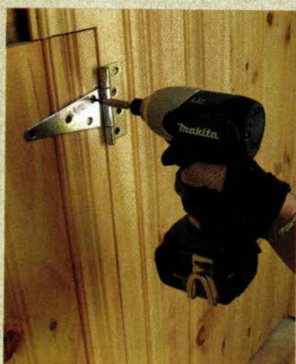
Install the door blanks using steel strap hinges, leaving about 1/8" gap at the jamb to allow room for the door to travel.
