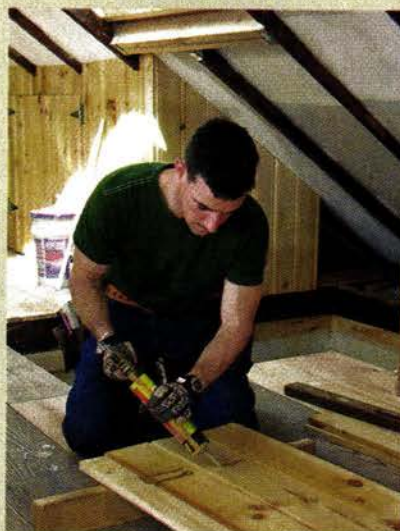
Square a line, dab some construction adhesive, and place the 1x4 rail (rails should be 2" shorter than door width) on the line.
