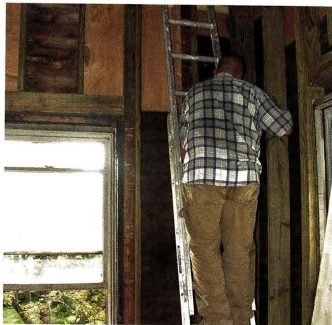
Installing new framing and sistering beams were critical to shoring up the tower.
