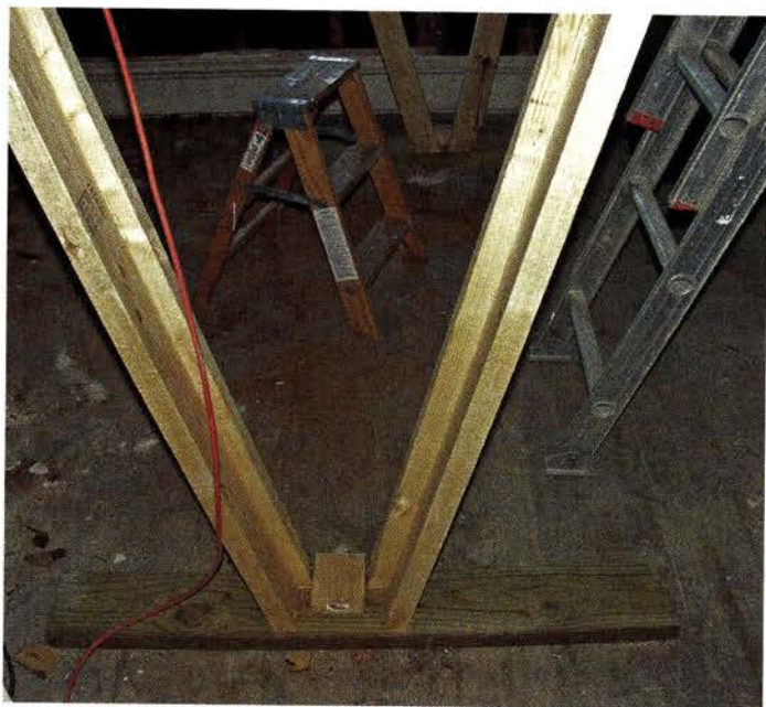
During the work, V-shaped supports propped up lateral temporary shoring; the system was moved daily to access new work areas.
