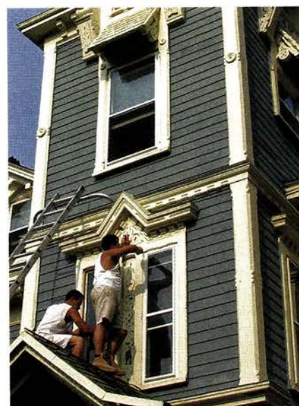
Craftsmen stripped and painted exterior decorative elements, and restored windows.
