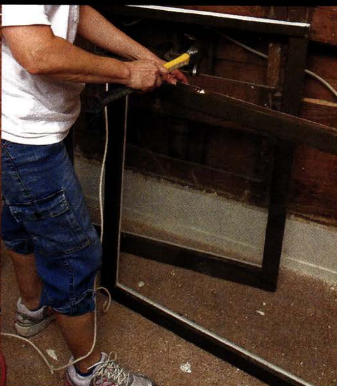
Pam nestles sash rope into an existing hole, then hammers it in place. The length of the rope fits into a routed channel along the sash.
