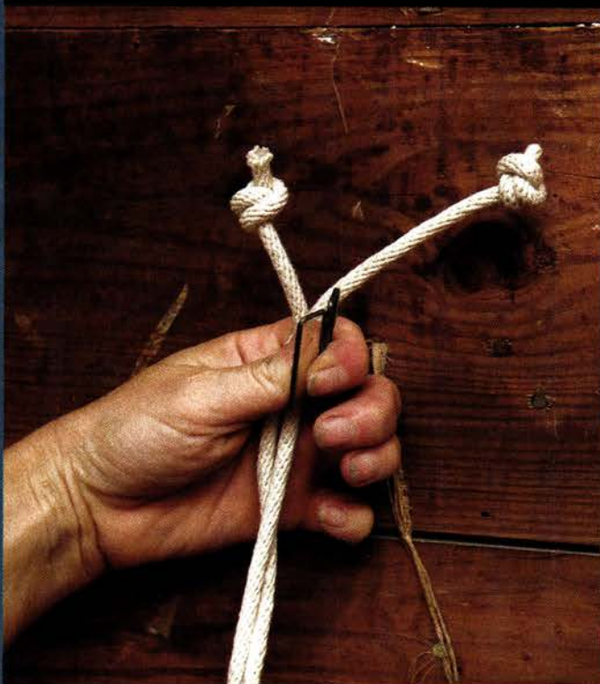
To attach sash rope securely, Pam prefers to use staples ("my insurance package," she says) in addition to nails.
