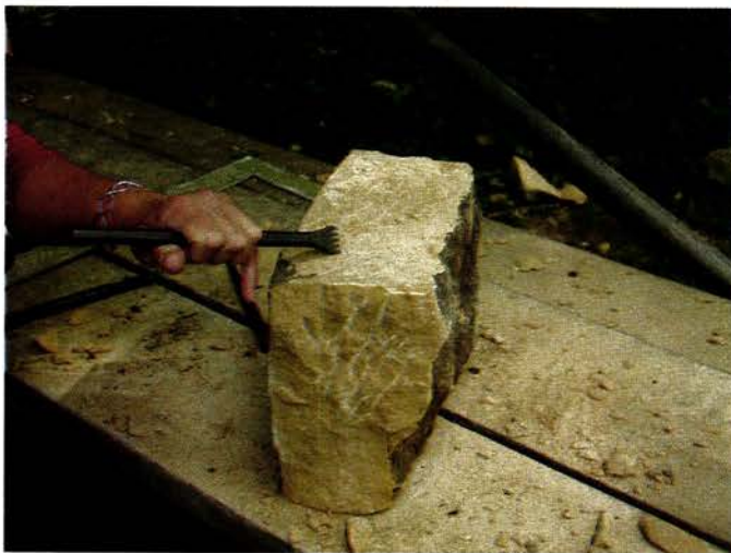
Use the tooth chisel to smooth high points on the stone's side surfaces for an easy fit into the wall cavity.
