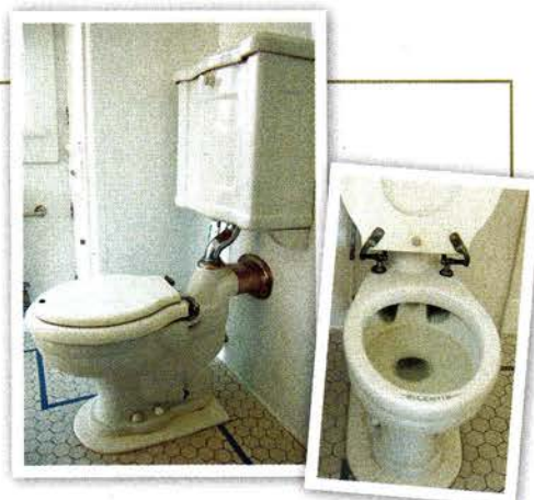
The early 20th-century bowl vent proved an ill-conceived attempt at sanitation.
