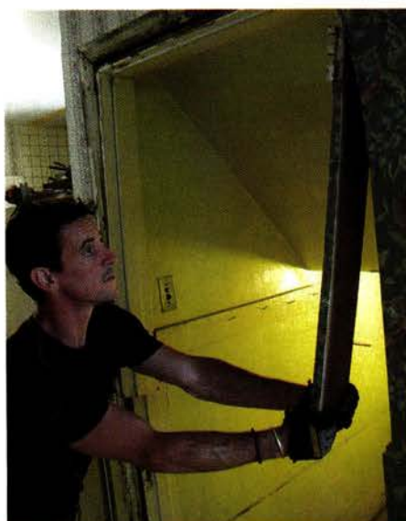
After taking a reciprocating saw to the old jamb and cutting the legs in half back to the framing, Mark wiggles the pieces out of the opening. Next, he works on getting the 4-light door ready for the new opening, using a framing square to identify areas that need a trim.
