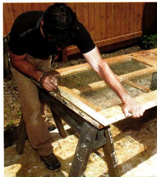
After taking a reciprocating saw to the old jamb and cutting the legs in half back to the framing, Mark wiggles the pieces out of the opening. Next, he works on getting the 4-light door ready for the new opening, using a framing square to identify areas that need a trim.
