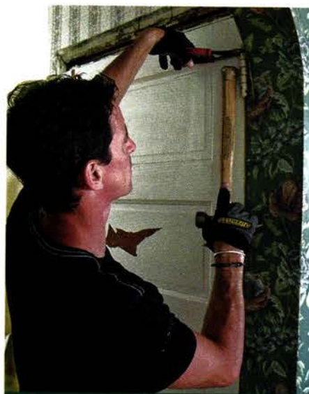
To move the home's four-light original back door to a new location atop the cellar stairs, Mark starts by removing the basement door's casings and using wire cutters to loosen the hinge bolts. Next, he lifts the old door out of the way.
