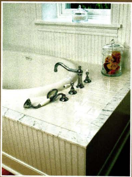
ABOVE: Because the marble pieces used for edging on the tub surround were so long and thin, Home Tech embedded them with steel rods to prevent cracking.
