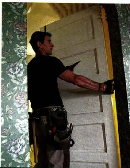
To move the home's four-light original back door to a new location atop the cellar stairs, Mark starts by removing the basement door's casings and using wire cutters to loosen the hinge bolts. Next, he lifts the old door out of the way.
