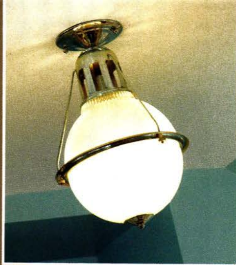
LEFT: The bathroom's distinctive overhead light is a vintage Holophane fixture augmented on the bottom with a dome-shaped diffuser to create what appears to be a cohesive sphere.
