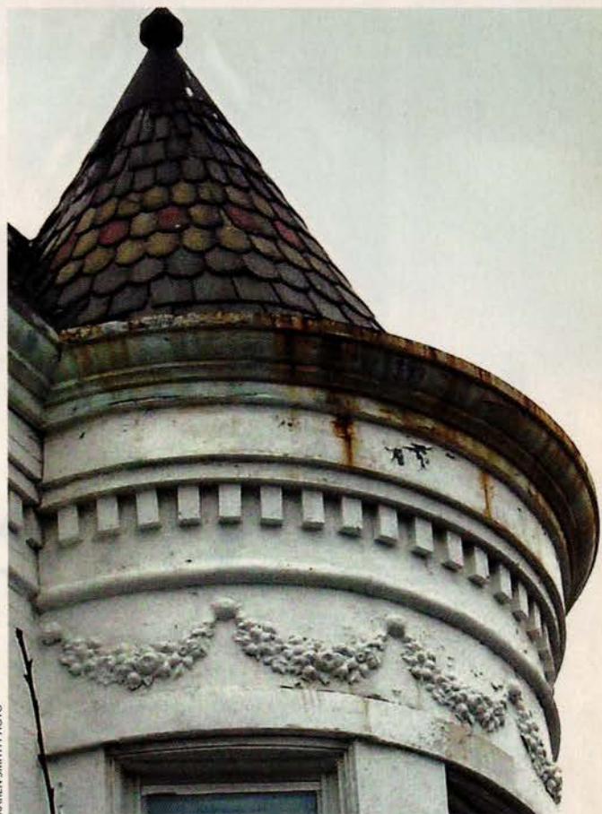
ABOVE: Mixing unlike metals will result in galvanic corrosion and telltale staining. BELOW: Bad design has ruined many an otherwise good repair, as in this example of a replaced wooden window sill that neglected to pitch away from the building, trapping water (and inviting rot) instead.
