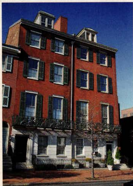
TOP: The projecting pent eave between floors and the plain doorway on the 1758 Rhoads-Barclay house are typical of earlier homes.
