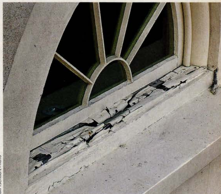
ABOVE: Mixing unlike metals will result in galvanic corrosion and telltale staining. BELOW: Bad design has ruined many an otherwise good repair, as in this example of a replaced wooden window sill that neglected to pitch away from the building, trapping water (and inviting rot) instead.
