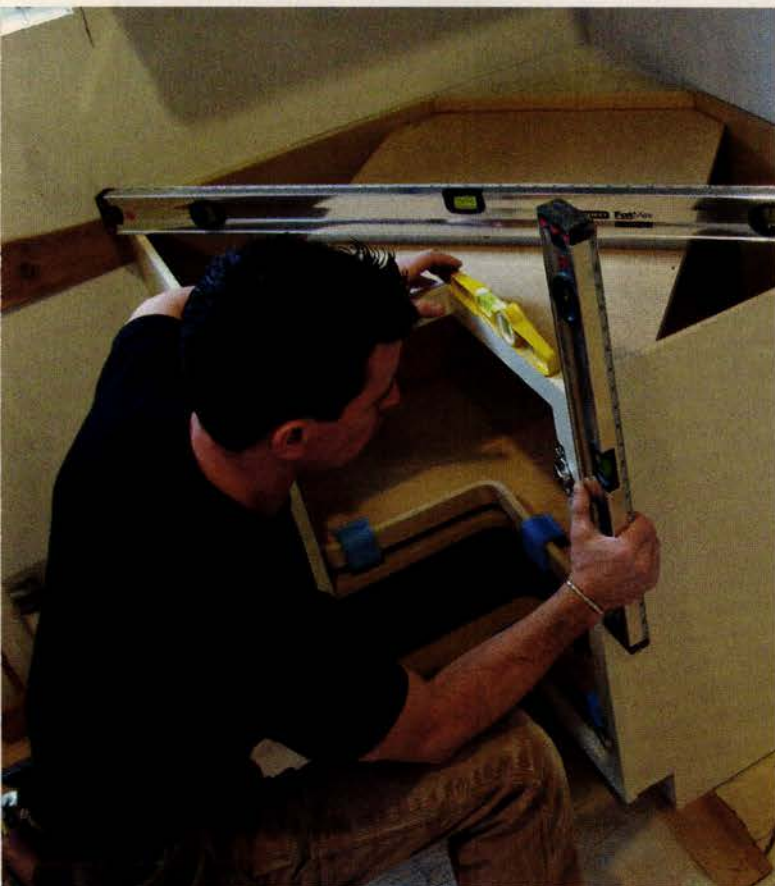
ABOVE: It's important to ensure that the cabinets are level and plumb in all directions. To guarantee that this is the case, Mark carefully checks all of the surfaces using a torpedo, a 2' level, and a 4' level consecutively. Then he double-checks it.
