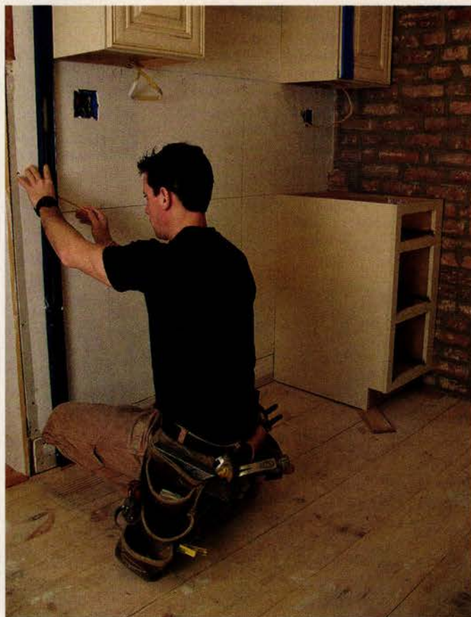
ABOVE: Base cabinets need to align with the uppers completely. Here, Mark plumbs down from the installed upper cabinet to line up the position of a stand-alone base. The stove will sit between this base and the corner unit, so he also measures the front opening to be certain it will fit.
