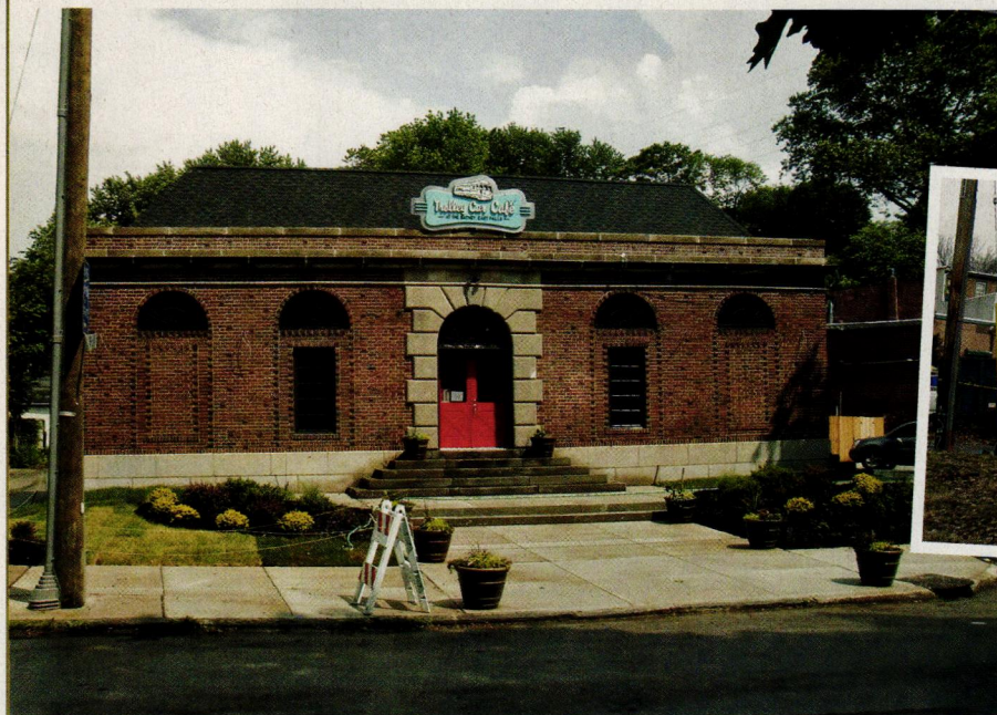
Work by a recent lessee, the Trolley Car Café (left), restored the missing hipped roof (below) on a building that was once a public bathhouse.
