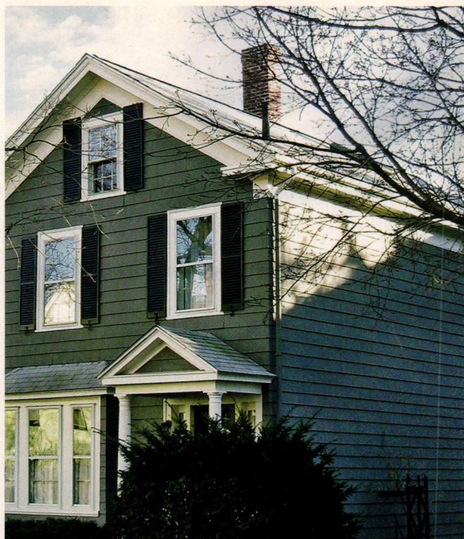
The unlined brick chimney on the Friedman-Sorenson's 1860 Greek Revival worker's cottage was degrading—eaten away by years of acidic exhaust from the boiler that was being vented through it. Consequently, before the project, the fireplace could only safely hold lighted candles, and its brick mantel didn't match the home's architecture.
