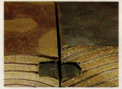
ABOVE: This over-sanded board (left) is worn away nearly through the top groove, making it prone to breakage.
