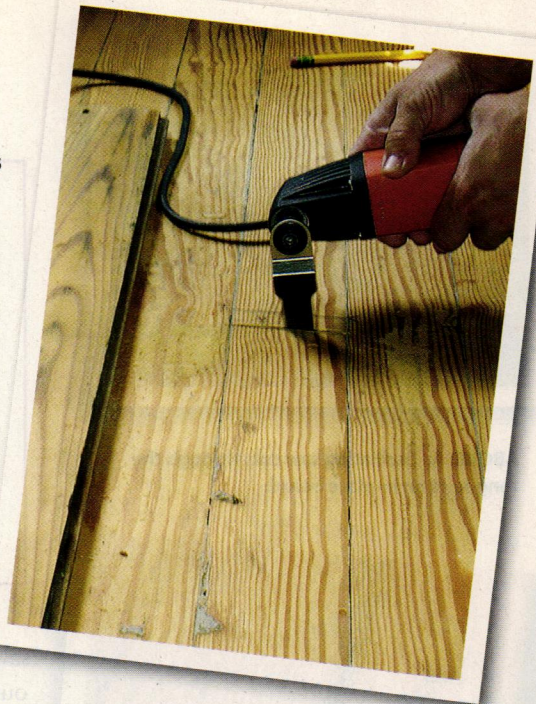
ABOVE: To replace a damaged floorboard, start by marking off the damaged material, then cutting it directly over the floor joist using an oscillating saw. You can then remove the damaged board.
