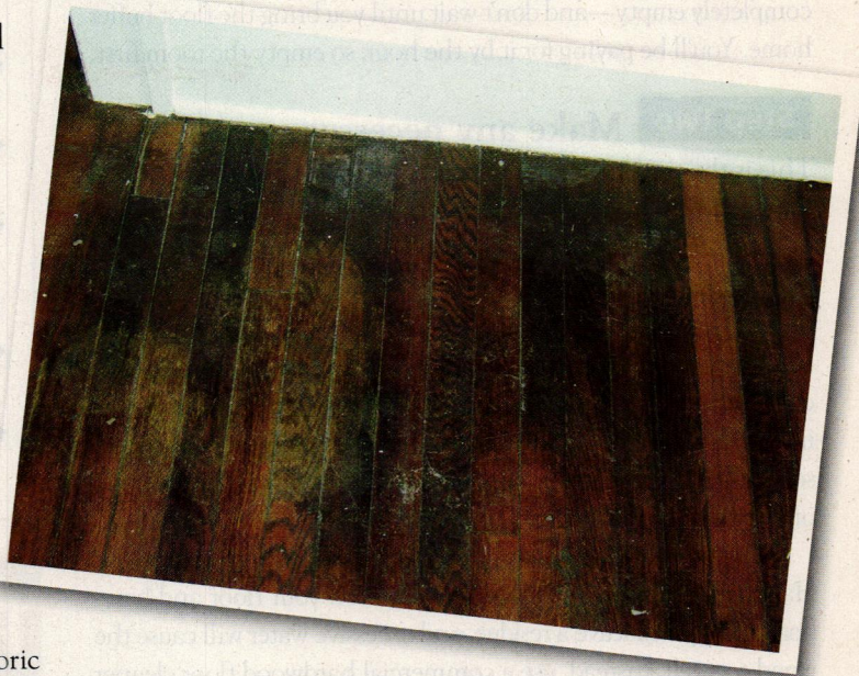
This room's scuffed-up hardwood flooring (above) looks good as new (opposite) after a simple recoating.
