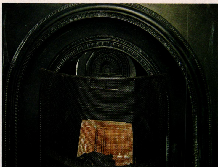
The new Victorian-style fireplace insert fit the space well, but its backplate didn't completely conceal the old brick. To create a seamless appearance, Charlie found a reclaimed wooden Greek Revival mantel and re-worked it, resizing its plinths and adjusting its height and depth to match the original molding and the built-in bookcase sitting beside it.
