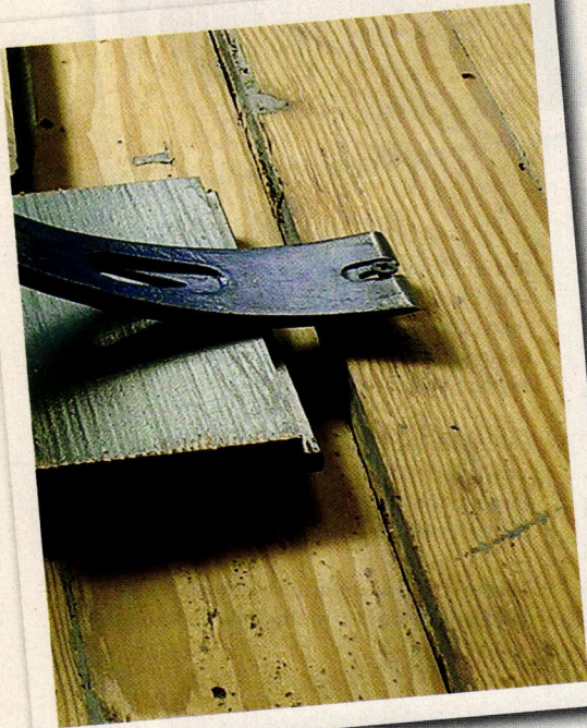
ABOVE: After cutting, remove damaged boards by attaching a screw and using a pry bar to gently lift them—a piece of wood beneath the bar helps avoid damaging neighboring boards. BELOW: Removing the replacement board's bottom groove lets it drop easily into place.
