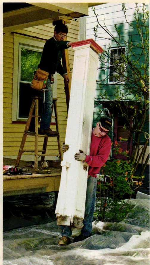
ABOVE: The old porch was crumbling away. In order to reconstruct it, Ted Robertson (left) and Mike Marini (right) began by spreading 6-mil plastic sheeting on the ground, bracing the porch's roof, then removing the columns. OPPOSITE: The new porch is not only picture-perfect, it's built to last, thanks to thoughtful structural details.
