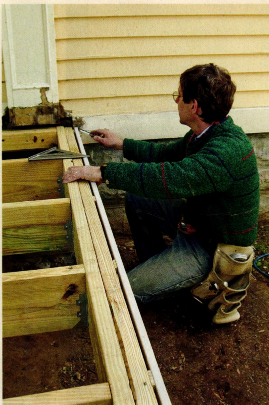
LEFT: Ted builds a new structural support from treated 2x8s. He starts by attaching a ledger to the wall with structural lag screws and pocketing the rim joists directly into original slots in the stone foundation. RIGHT: One of Ted's tricks for making porches that last is ensuring that parts have good ventilation; here, he accomplishes this by installing vertical shims between the exterior joist and the finish apron (the shims are visible in the gap between these two elements).
