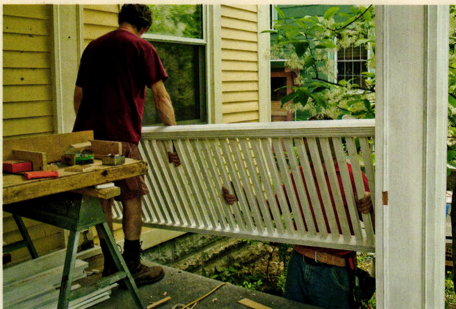
LEFT & BELOW: The men assembled the balustrade in the shop, then installed it as a single completed unit. To help the columns and posts last—by enabling air circulation and preventing trapped water—Ted rested them on thin lead shims before completing assembly.
