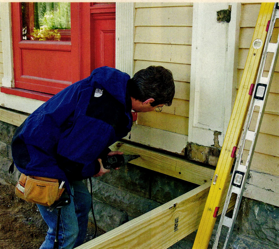
LEFT: Ted builds a new structural support from treated 2x8s. He starts by attaching a ledger to the wall with structural lag screws and pocketing the rim joists directly into original slots in the stone foundation. RIGHT: One of Ted's tricks for making porches that last is ensuring that parts have good ventilation; here, he accomplishes this by installing vertical shims between the exterior joist and the finish apron (the shims are visible in the gap between these two elements).
