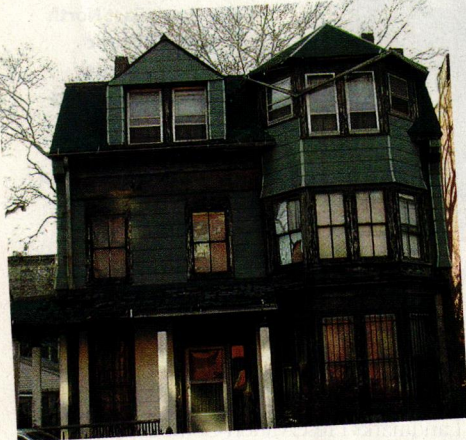
With the blessing of the New York City Landmarks Preservation Commission, the owners of this Victorian-era house in Brooklyn's Clinton Hill Historic District replaced modern composite shingle siding (left) with more appropriate white-painted cedar shingles. In areas where the slate roof had been replaced with asphalt shingles, the Commission allowed for in-kind replacement, but required the remaining slate roof to be maintained.
