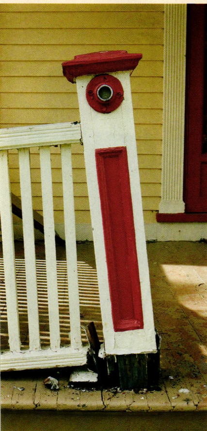
ABOVE: The old porch was crumbling away. In order to reconstruct it, Ted Robertson (left) and Mike Marini (right) began by spreading 6-mil plastic sheeting on the ground, bracing the porch's roof, then removing the columns. OPPOSITE: The new porch is not only picture-perfect, it's built to last, thanks to thoughtful structural details.
