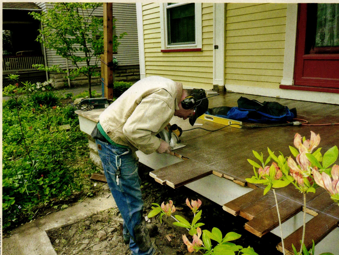
RIGHT: With the deck installed, the men pop a chalk line, then cut the end boards to a uniform length. Afterward, they use a router to finish off the edges.
