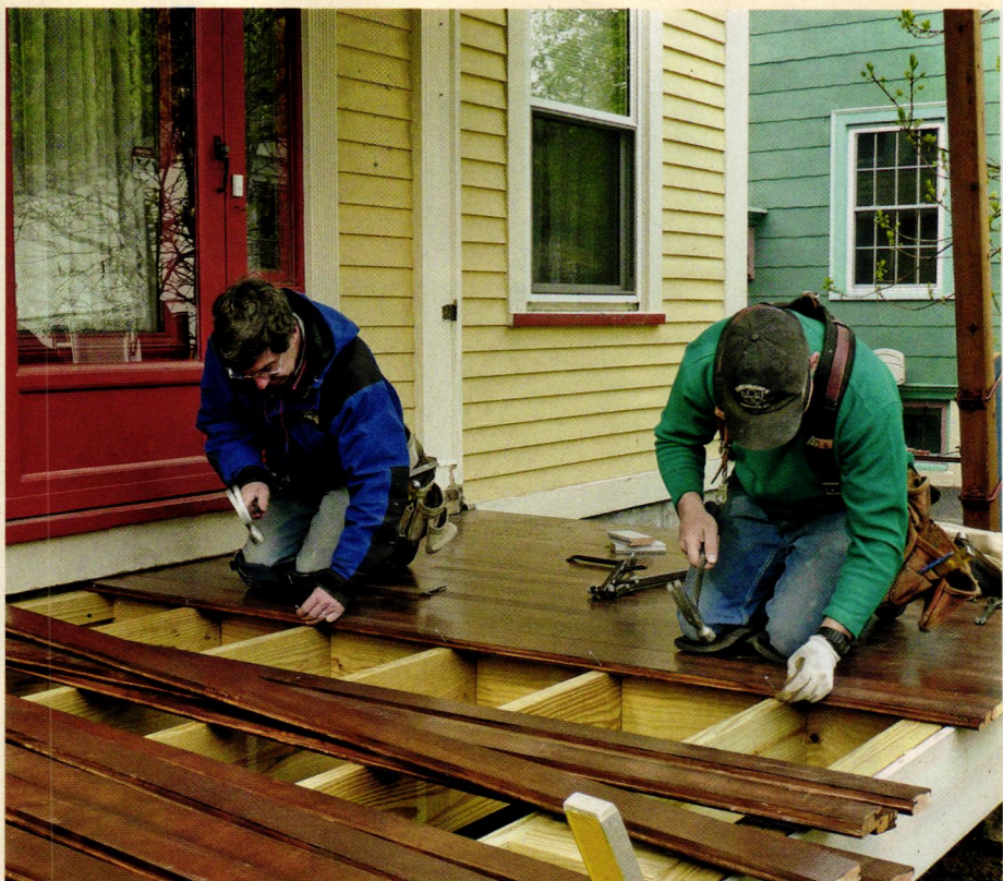
LEFT: Another of Ted's tricks for lasting porches: gluing the first and last three decking boards together with marine epoxy, a technique that helps keep the end boards from pulling apart. These three tongue-and-groove boards on sawhorses have just finished clamp time, and are ready to be installed. RIGHT: Ted and Mike blind-nail the rest of the decking boards into place.
