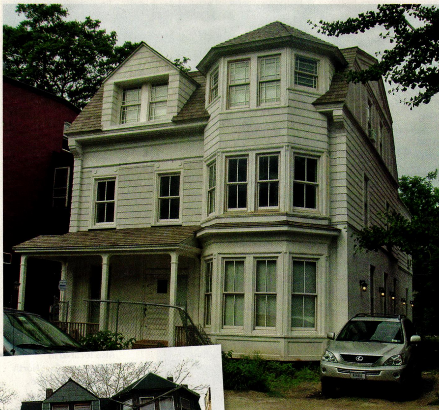
With the blessing of the New York City Landmarks Preservation Commission, the owners of this Victorian-era house in Brooklyn's Clinton Hill Historic District replaced modern composite shingle siding (left) with more appropriate white-painted cedar shingles. In areas where the slate roof had been replaced with asphalt shingles, the Commission allowed for in-kind replacement, but required the remaining slate roof to be maintained.
