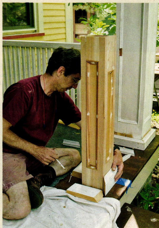
LEFT & BELOW: The men assembled the balustrade in the shop, then installed it as a single completed unit. To help the columns and posts last—by enabling air circulation and preventing trapped water—Ted rested them on thin lead shims before completing assembly.
