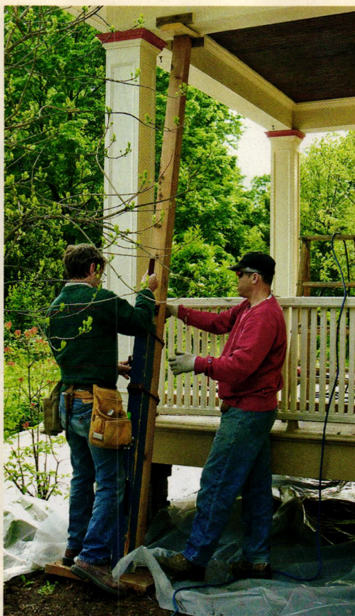
ABOVE: The old porch was crumbling away. In order to reconstruct it, Ted Robertson (left) and Mike Marini (right) began by spreading 6-mil plastic sheeting on the ground, bracing the porch's roof, then removing the columns. OPPOSITE: The new porch is not only picture-perfect, it's built to last, thanks to thoughtful structural details.
