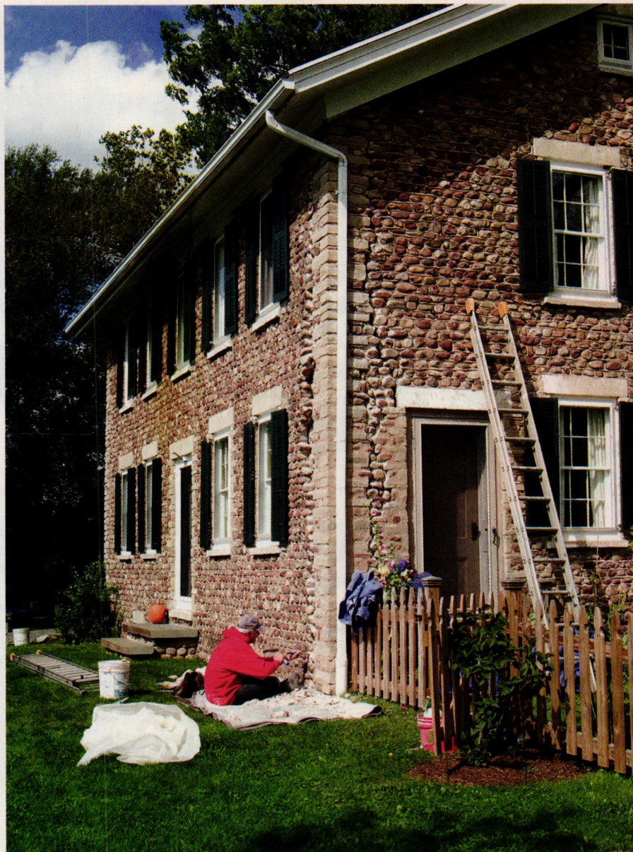
Improperly keyed quoins and years of inappropriate repairs had caused major cracking (visible above) on the corners of this cobblestone house in upstate New York. Stonemason Marty Naber restored the walls by removing old mortar and caulk and replacing it with new lime-based mortar. Today, the house (at left, with shutters removed to highlight the stonework) is good as new.
