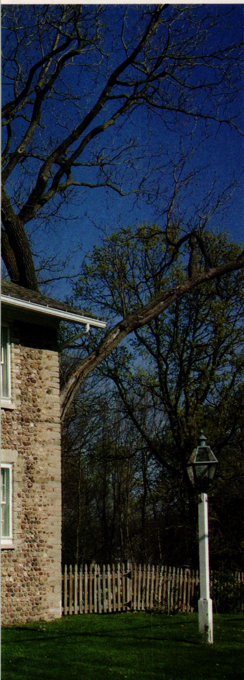
Improperly keyed quoins and years of inappropriate repairs had caused major cracking (visible above) on the corners of this cobblestone house in upstate New York. Stonemason Marty Naber restored the walls by removing old mortar and caulk and replacing it with new lime-based mortar. Today, the house (at left, with shutters removed to highlight the stonework) is good as new.
