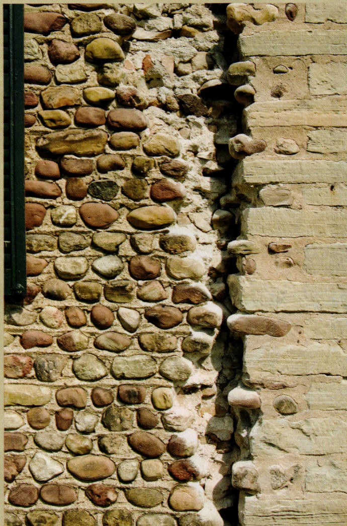
Once the old mortar and inappropriate repair materials were completely removed (left), Marty filled in the wall with new rubble stone and mortar, then returned the original cobblestones to the wall (above).
