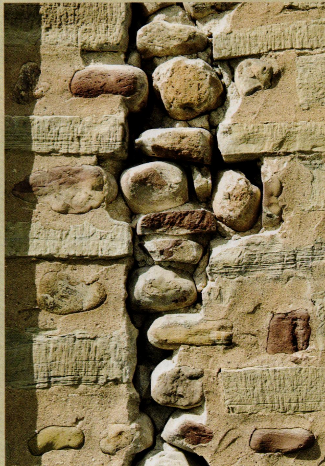
Once the old mortar and inappropriate repair materials were completely removed (left), Marty filled in the wall with new rubble stone and mortar, then returned the original cobblestones to the wall (above).
