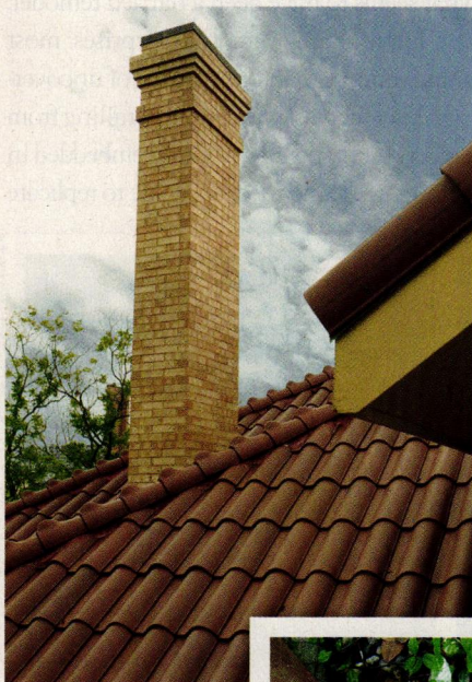
Tile fragments excavated in the garden confirmed the original roof's manufacturer—Ludowici—who was able to provide a perfect match.
