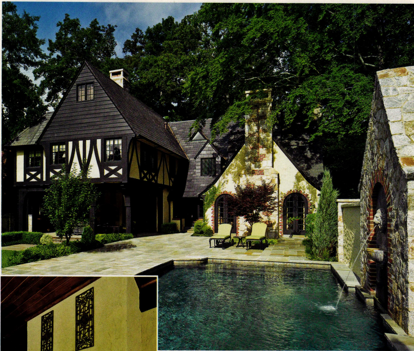
ABOVE: The overhang of the second-floor master suite addition (at left) allowed for a new covered terrace housing an outdoor kitchen. New half-timbering is cypress instead of pine, but was carefully cut and painted to match the original trim.
