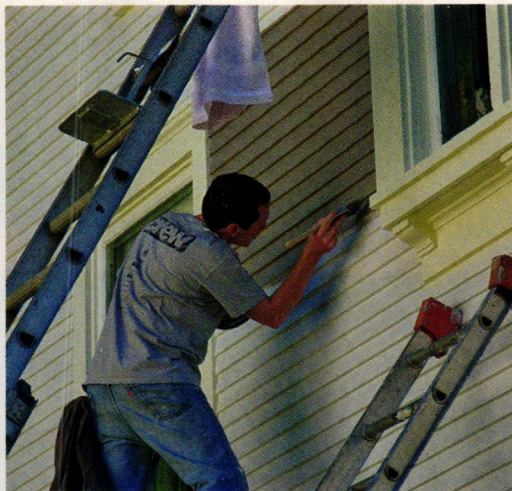
After using carbide scrapers, the wood was very clean (far left); also visible are nails primed with a rust inhibitor. Ryan carefully applies a coat of finish paint (near left).
