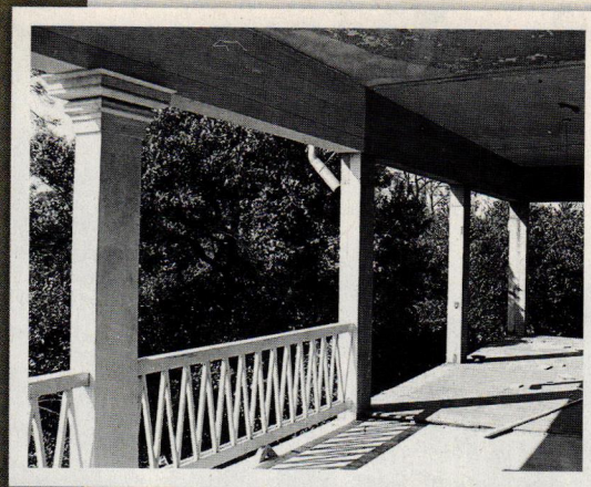
LEFT & ABOVE: Historic photos guided the rebuilding of the stacked-wood column capitals, similar to those on other 1850s houses in the area.
