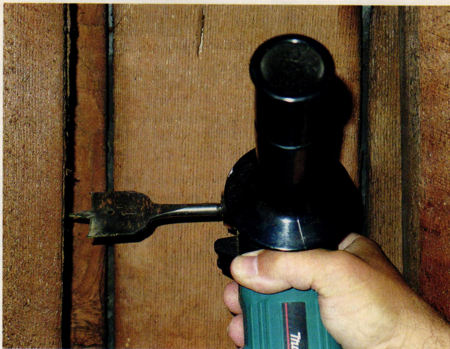
A right angle drill fits easily into the space between wall studs.
