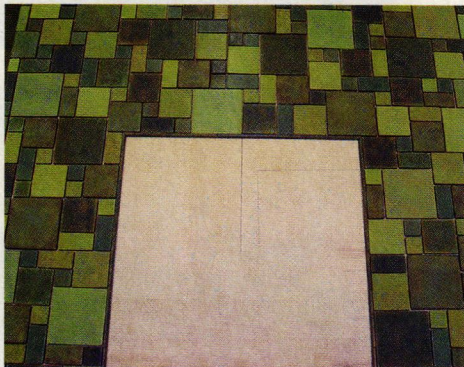
The new facing uses handmade Syzygy tiles; Michelle laid the pattern out on the floor first to finesse the color distribution and grout lines.
