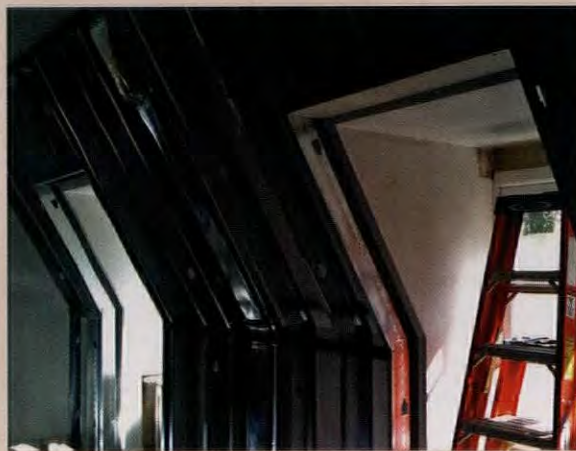
LEFT TO RIGHT: In one of the children's rooms, a false wall was built to disguise the ductwork. The far left photo shows the ducts attached to the wall; the center photos show the wall in various stages of completion. At far right, the new wall assembly is highlighted with a cheerful, contrasting paint scheme.
