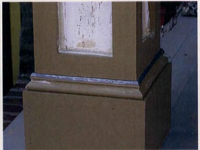
ABOVE: When joints at the base of square columns point downward and are protected by flashing, rainwater naturally slides off the wooden element, preventing infiltration that can lead to rot.
