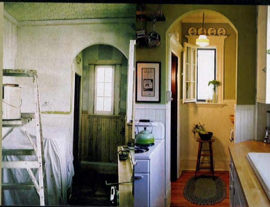
LEFT: The dimensions for the new passageway between the kitchen and pantry were based on a ghost Ryan and Montana found under the carpet. RIGHT: With beadboard wainscoting and a reproduction light fixture, the new butler's pantry pays homage to the original space.
