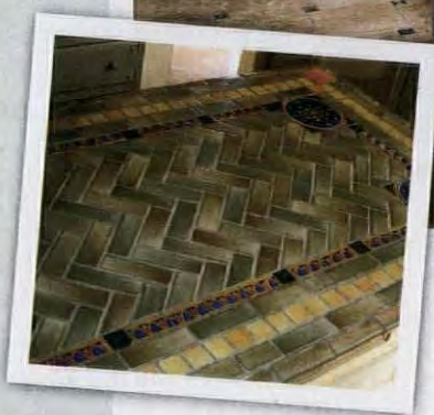
LEFT & ABOVE: The edging for the island was the easiest part, says Judy; the 5¾" x 2½" cornice tiles are designed to curve around the counter's edge. Cutting the angles of the herringbone tile freehand proved to be the biggest challenge.
