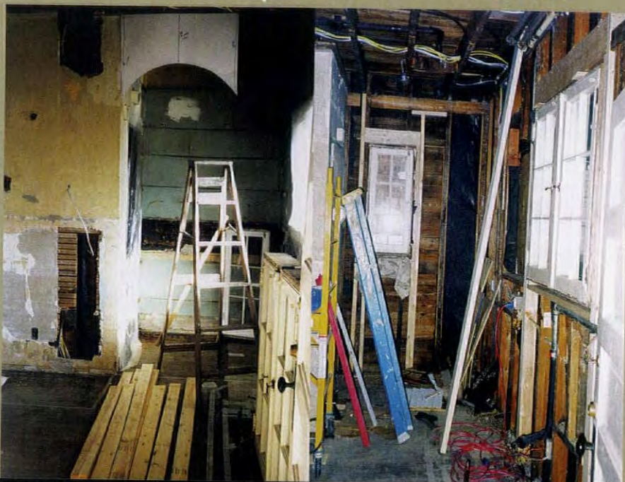
LEFT: Upon dismantling the kitchen, Ryan and Montana found ghosts of original butler's pantry shelving (visible on the back wall below a mock-up of the new passageway). RIGHT: The layout of the pantry was reconfigured to add a salvaged casement window to bring in additional light.
