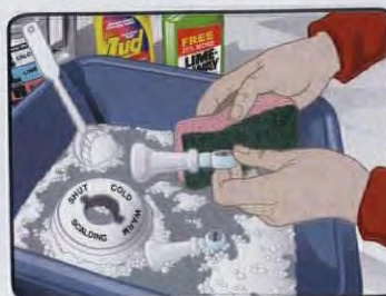
LEFT TO RIGHT: To clean up vintage fixtures, you'll need a basin, scrub brush and sponge, some CLR or Lime-Away, and Zud. Soak the part in a mixture of water and one of the first two cleaners, then brush it down and follow up with Zud on the scrubber. Rinse well.
