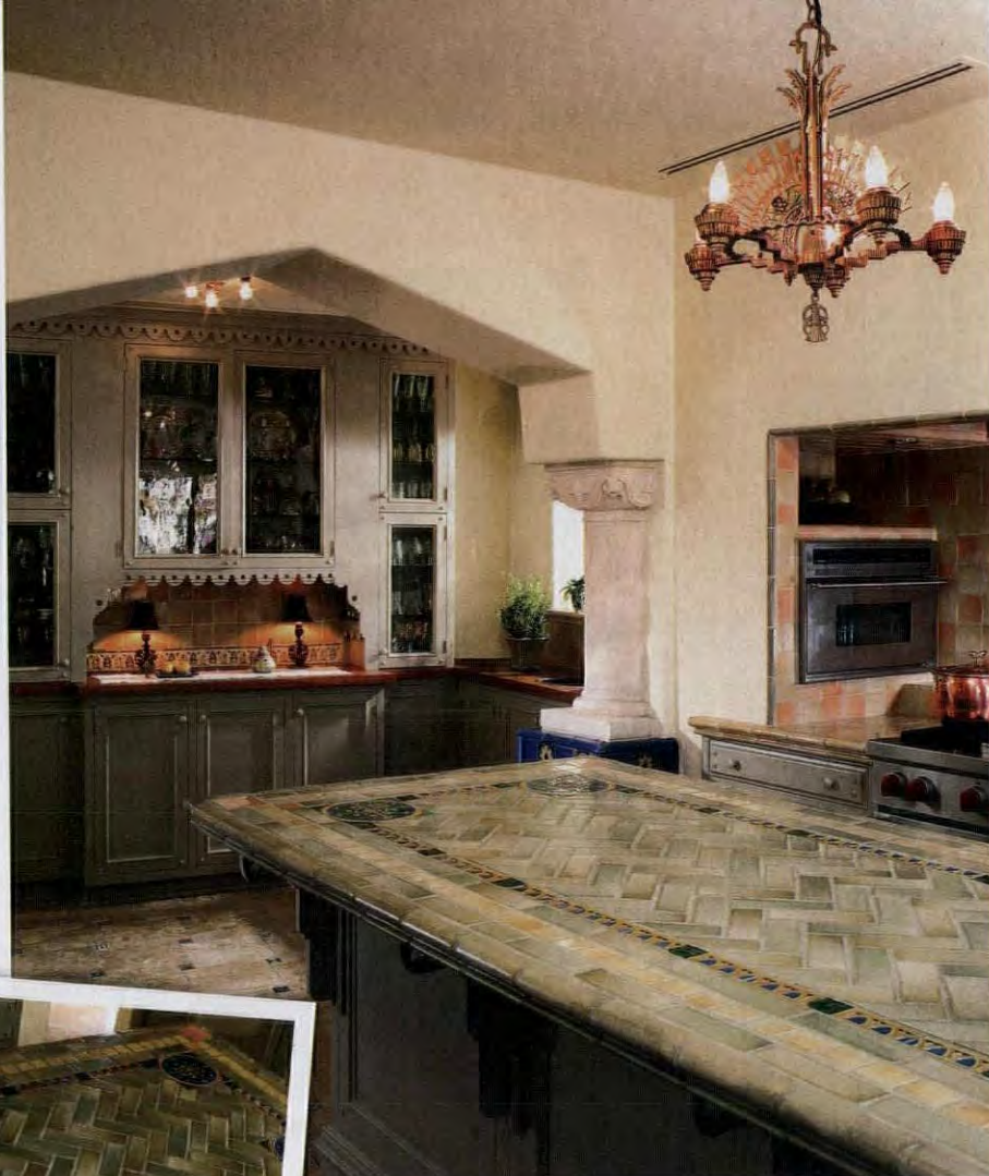
LEFT & ABOVE: The edging for the island was the easiest part, says Judy; the 5¾" x 2½" cornice tiles are designed to curve around the counter's edge. Cutting the angles of the herringbone tile freehand proved to be the biggest challenge.
