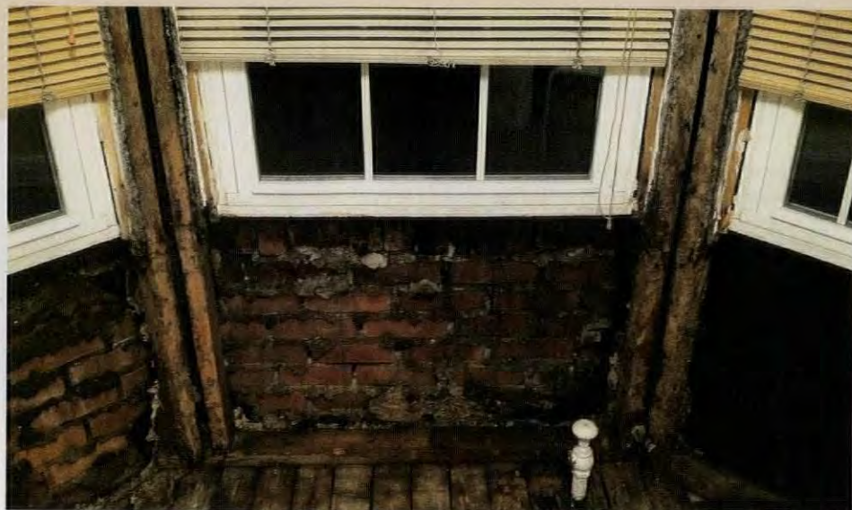
ABOVE: Termites invaded the wood framing around this reader’s bay window, eating away at the wood (left). Often, damaged members can be joined to new wood, which will strengthen them while avoiding the hassle of complete replacement.
