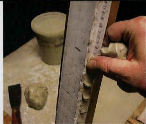
A solid "bed" of putty in the sash's glazing rabbets helps seat the pane of glass.
