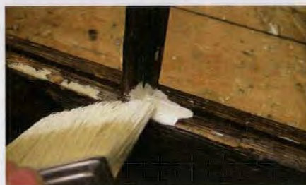
Puddling the primer at each joint helps it soak in and seal the end-grain.
