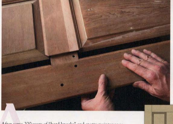
OPPOSITE: Six-panel doors are common on Federal, Georgian, and Colonial Revival houses, such as this 1938 Colonial Revival on Cape Cod. LEFT: Repairs often require disassembling and reassembling the door.
