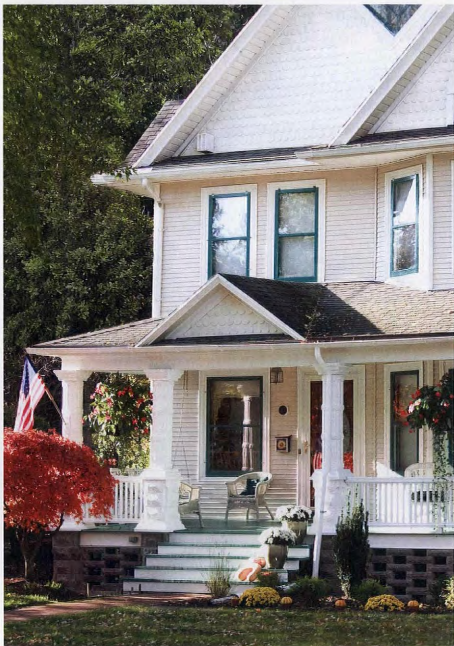
ABOVE: The restored porch—with new concrete blocks—is ready to weather another century.
