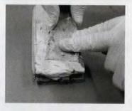
Press the epoxy filler into the defect with your fingers, then use a flexible putty knife to apply enough pressure to force the epoxy into all of the crevices. This type of epoxy can be difficult to smooth, but it is easy to sand. Build it higher than the surface and sand to match the surrounding wood.
