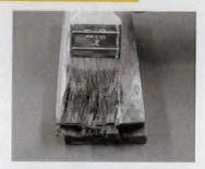
Before you apply an epoxy filler, prepare the surface with a consolidant from the same manufacturer. A consolidant is a thinned form of epoxy that soaks into the remaining compromised wood fibers and improves the bonding surface for the filler that follows.
