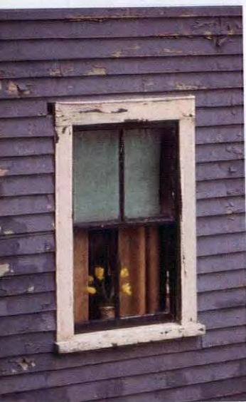
Even when you know that moisture is the cause of peeling paint, it can be difficult to find the water incursion or source of condensation.
