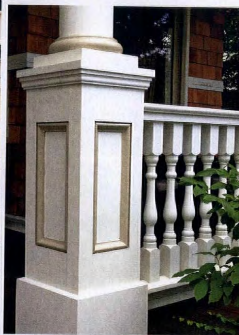
FROM TOP: A new "snowflake" balustrade on an Italianate is the finishing touch for the fully restored front porch. A new balustrade turned in Port Orford cedar by Western Spindle returns period detail to a restored porch. Even fancy-cut porch elements can survive if they're kept painted—this balustrade dates to 1890.
