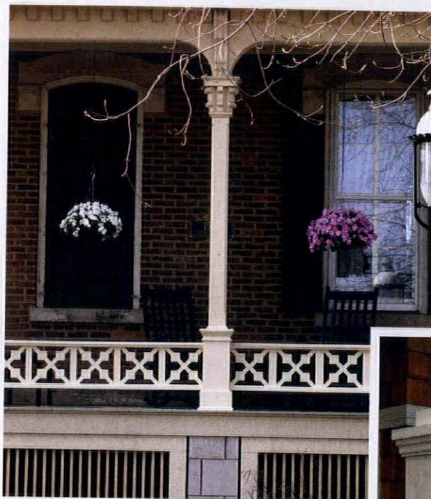
FROM TOP: A new "snowflake" balustrade on an Italianate is the finishing touch for the fully restored front porch. A new balustrade turned in Port Orford cedar by Western Spindle returns period detail to a restored porch. Even fancy-cut porch elements can survive if they're kept painted—this balustrade dates to 1890.
