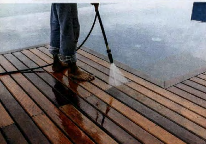
TOP: Applying stain or sealer with a sponge mop will save your knees. ABOVE: Use low pressure (1200 to 1500 psi) to clean a deck.
