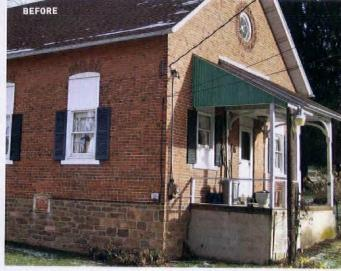
The tall schoolhouse windows had been removed. replaced with small vinyl windows. The makeover included installation of eight newly milled windows. The enlarged stoop was restored to its original configuration, with steps on either side of the main door. The exterior brick required only minor cleaning and pointing. BELOW: Donna and her husband got to know neighbors and local lore through their restoration.
